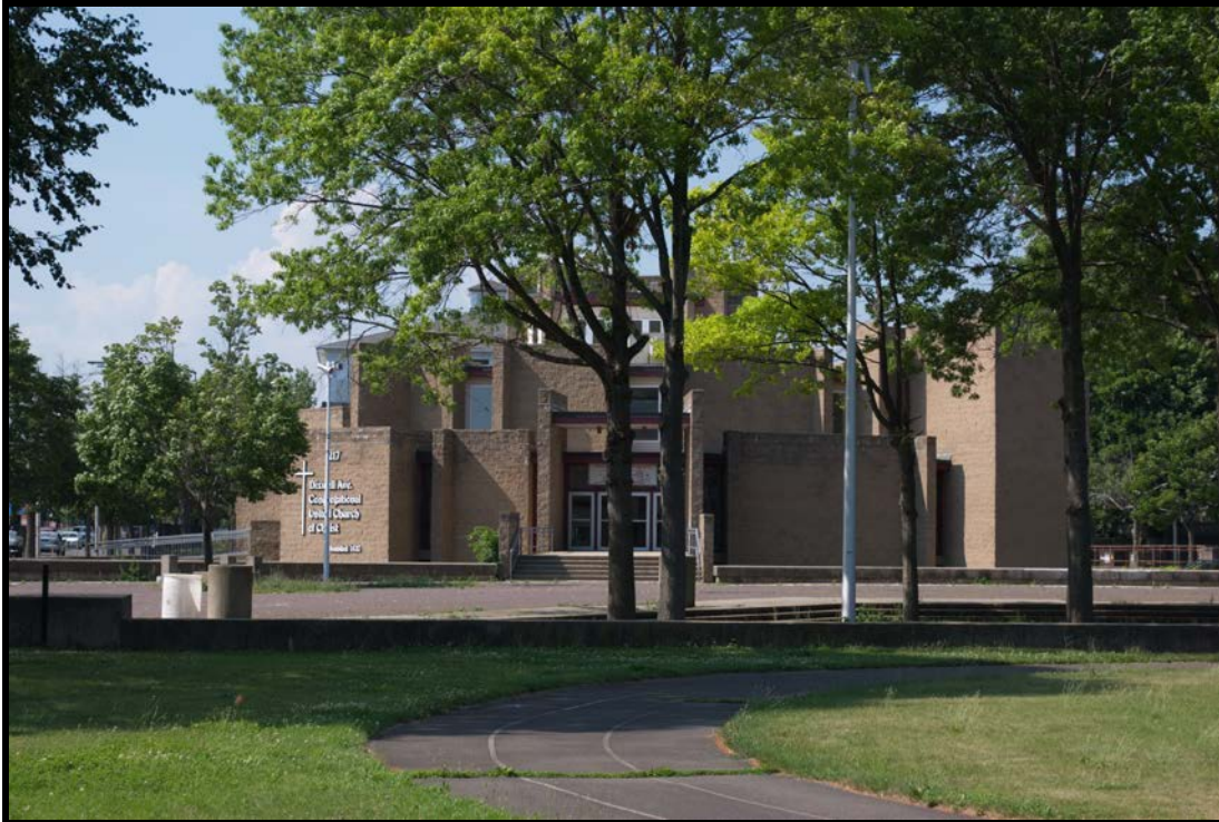
Photograph #5 of 31: South elevation. Camera facing N.
