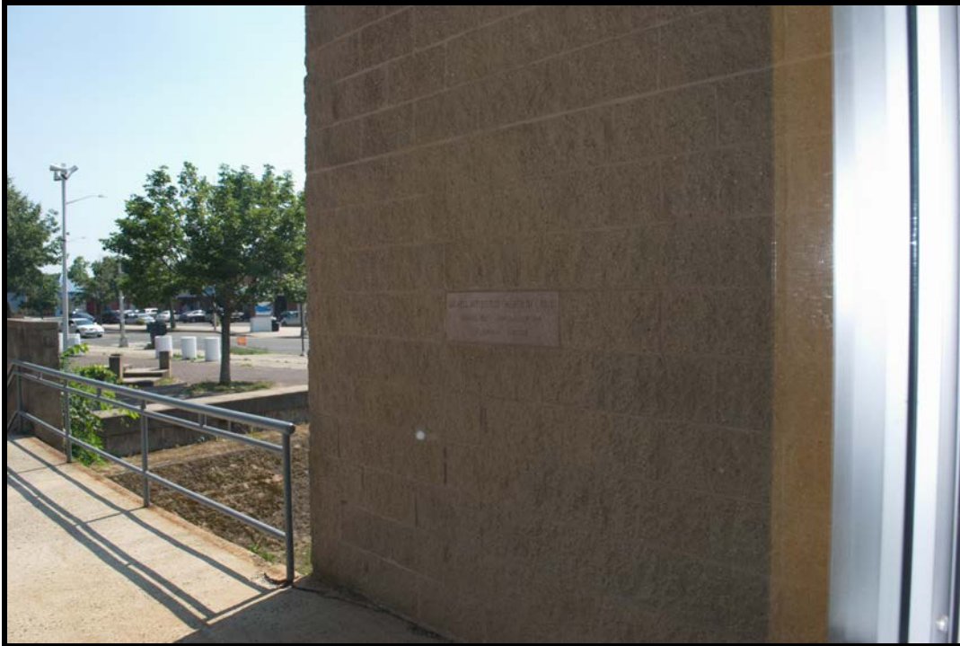
Photograph #23 of 31: Exterior detail. Camera facing SW.
