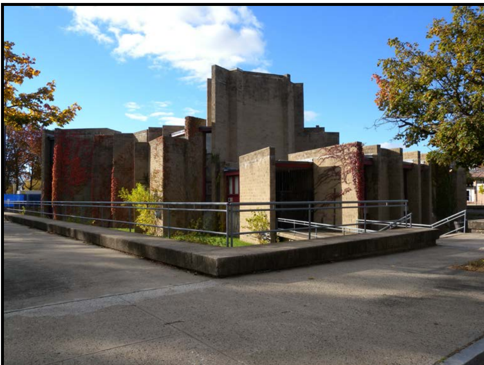
Photograph #10 of 31: Northwest elevation. Camera facing SE.
