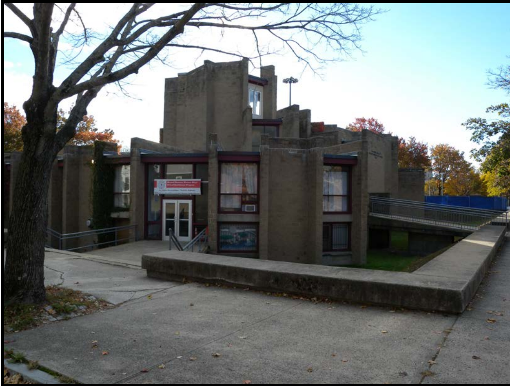
Photograph #11 of 31 Northwest elevation. Camera facing SE.
