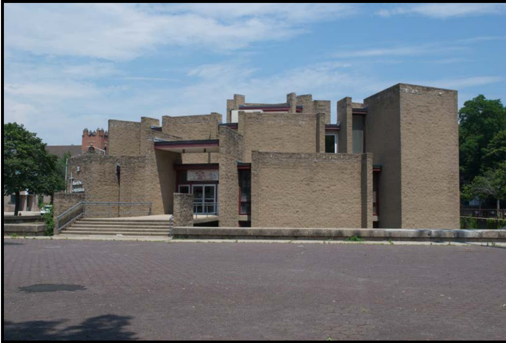
Photograph #7 of 31: Southeast elevation. Camera facing NW.
