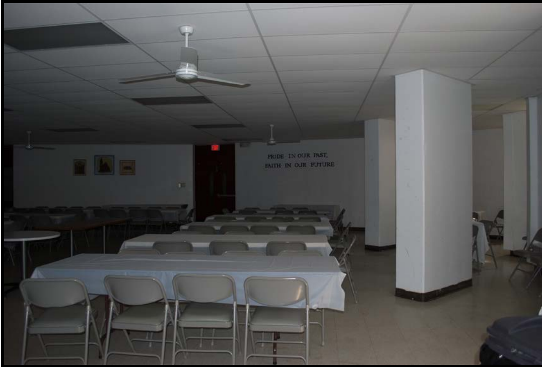
Photograph #30 of 31: Interior, lower level assembly hall. Camera facing N.
