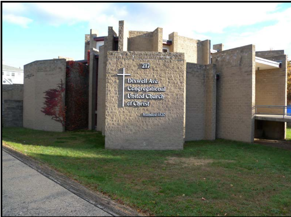
Photograph #8 of 31: Exterior detail. Camera facing NE.
