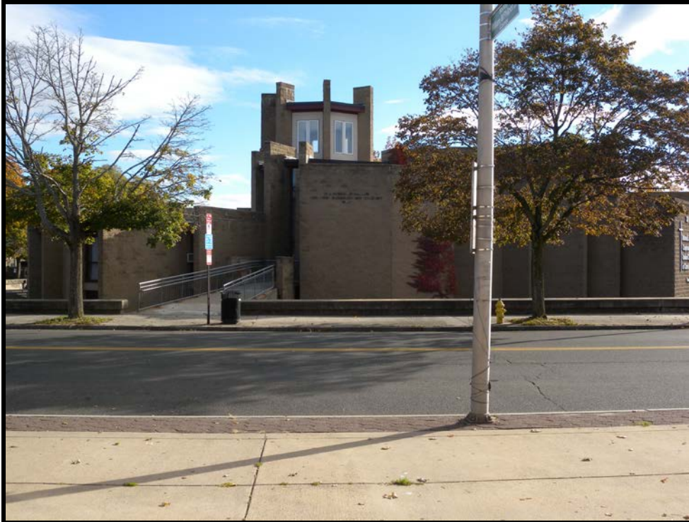
Photograph #9 of 31. West elevation. Camera facing E.
