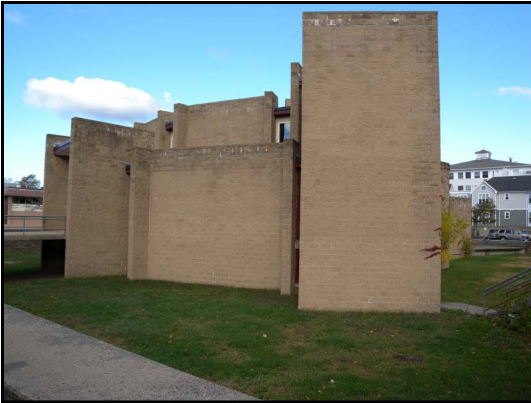
Photograph #14 of 31: Exterior detail. Camera facing NW.
