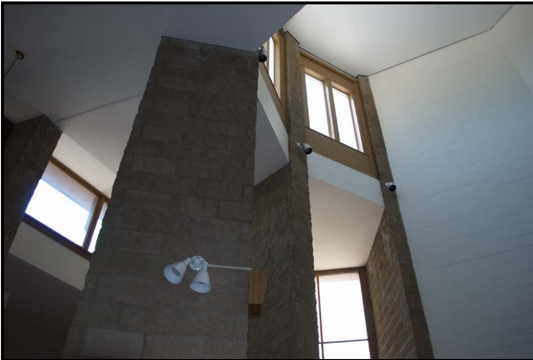
Photograph #26 of 31: Interior window detail, main worship area. Camera facing NW.
