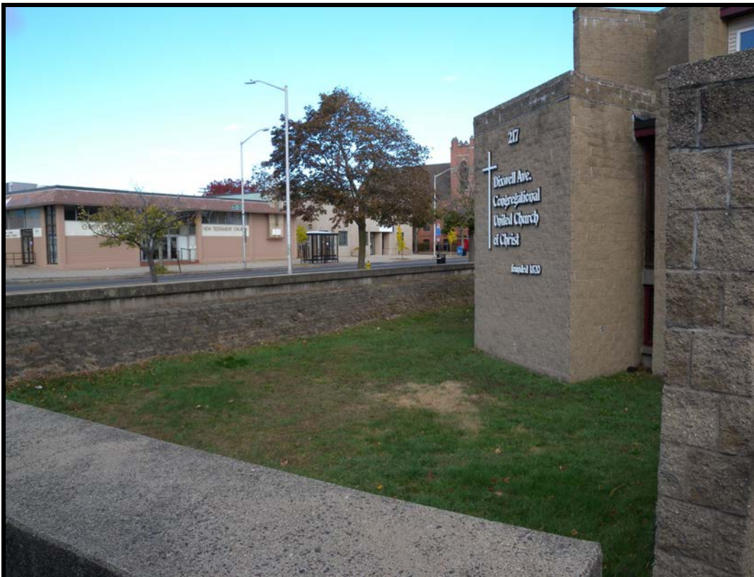
Photograph #24 of 31: Exterior detail. Camera facing NW.
