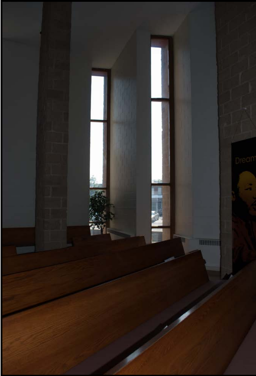
Photograph #28 of 31: Interior, nave window detail. Camera facing SW.
