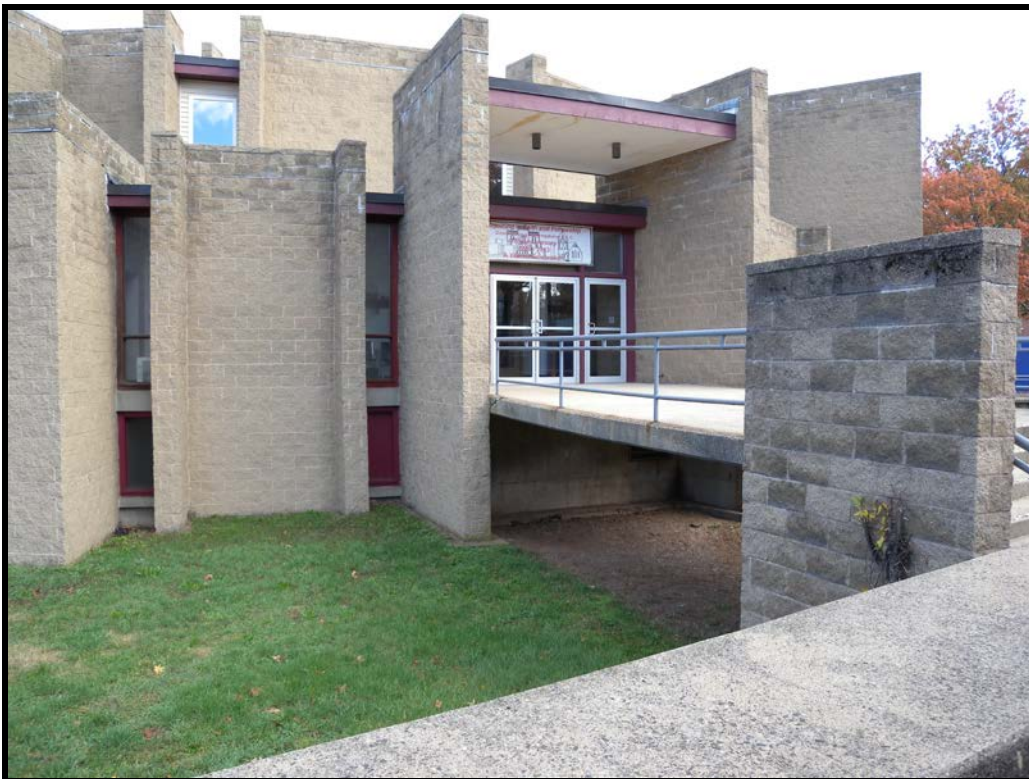
Photograph #16 of 31: South entrance. Camera facing NE.
