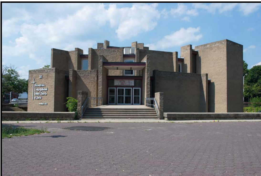
Photograph #6 of 31: South elevation. Camera facing N.
