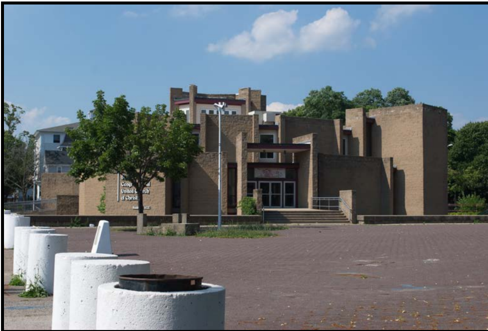
Photograph #4 of 31: Southwest elevation. Camera looking NE.
