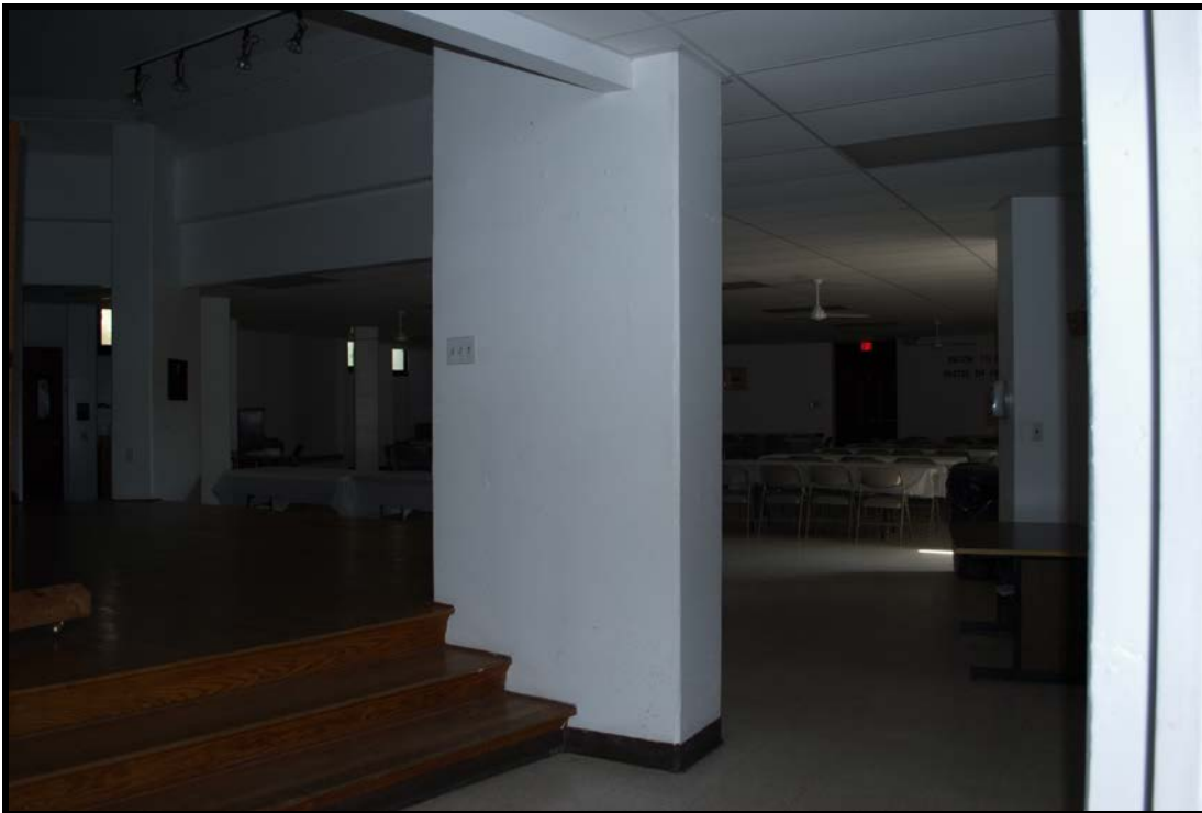
Photograph #31 of 31: Interior pier detail, lower level. Camera facing NE.
