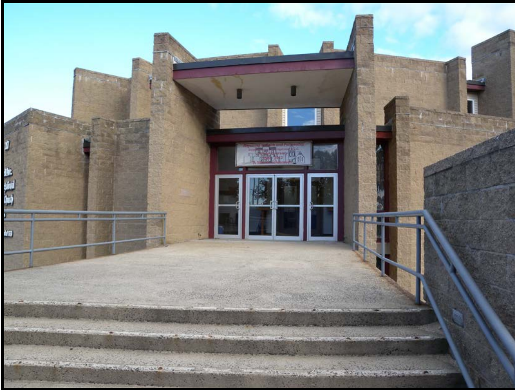
Photograph #15 of 31: South entrance. Camera facing N.
