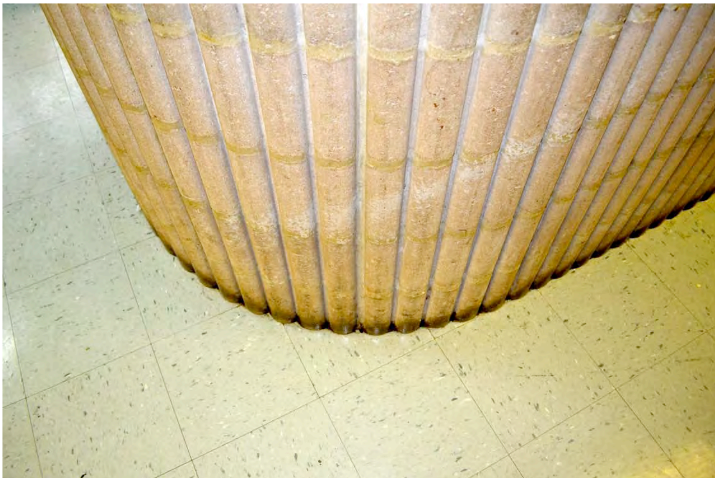
Detail of typical upper-floor corridor wall, showing ribbed concrete block details. Camera facing northeast. Photograph 19 of 19.
