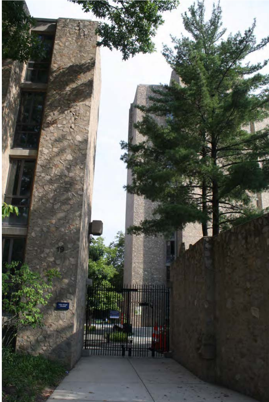
Photo 8. North view of the entry to Stiles College from Tower Parkway; camera facing south.
