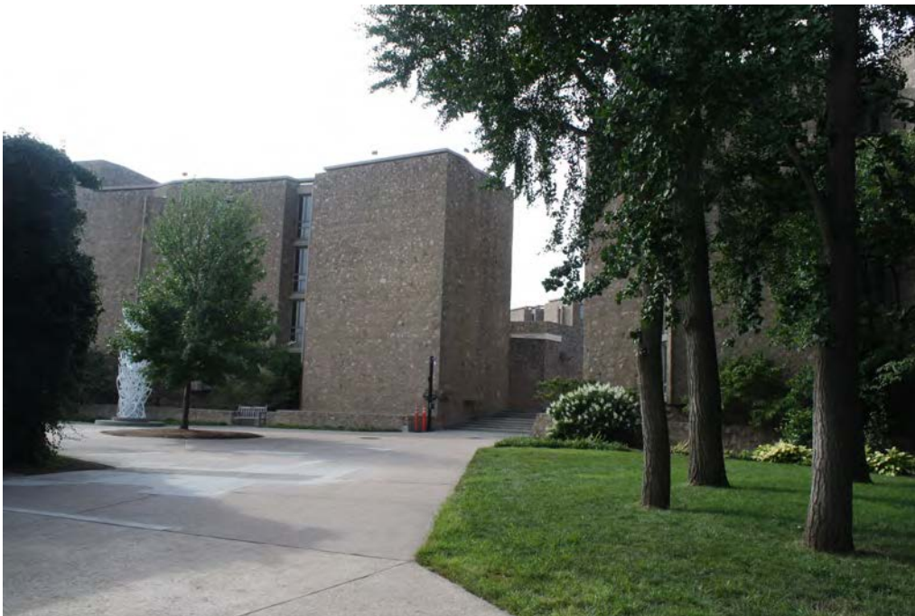
Photo 15. South view of the walk between Stiles (left) and Morse (right) Colleges; camera facing north.
