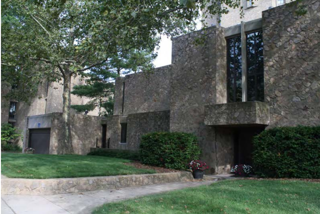
Photo 9. North view of the Stiles College Master's House from Tower Parkway; camera facing southeast.
