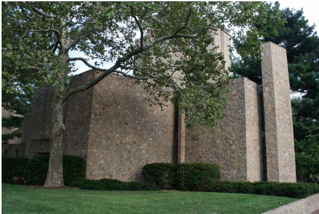
Photo 10. Northwest view of the Stiles College Master's House from Broadway; camera facing east.
