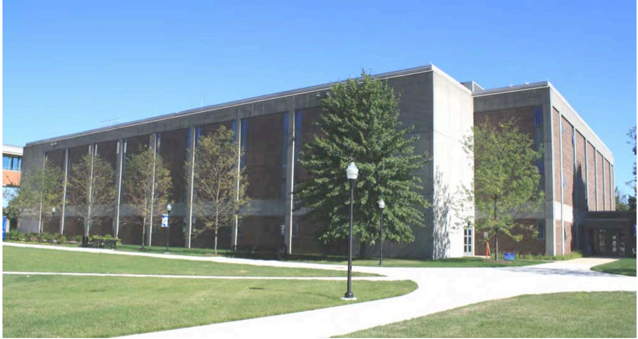
Photo 3. Southwest view of Jennings Hall, camera facing northeast.
