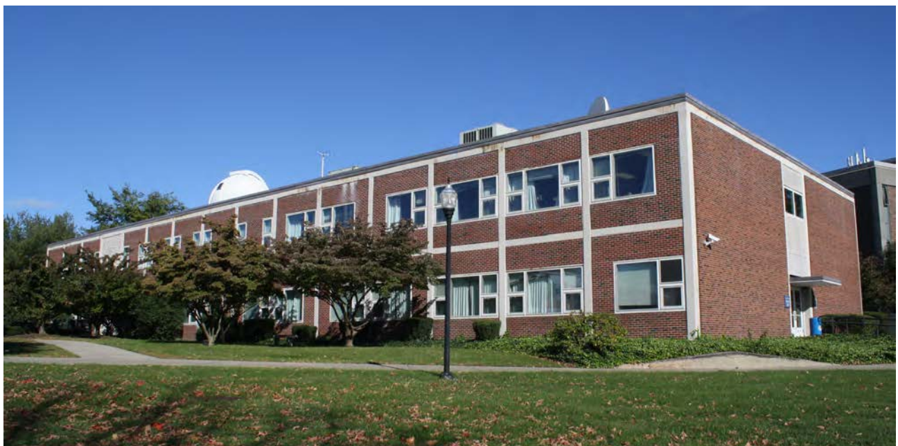
Photo 4. Southeast view of Morrill Hall, camera facing northwest.
