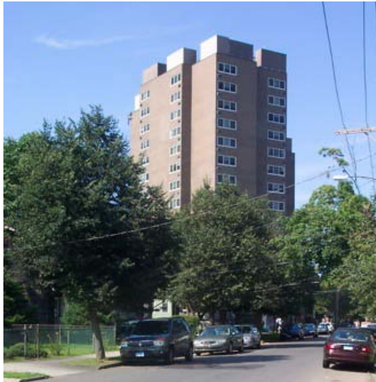
1. Northeast view from Bristol Street, camera facing southwest.
