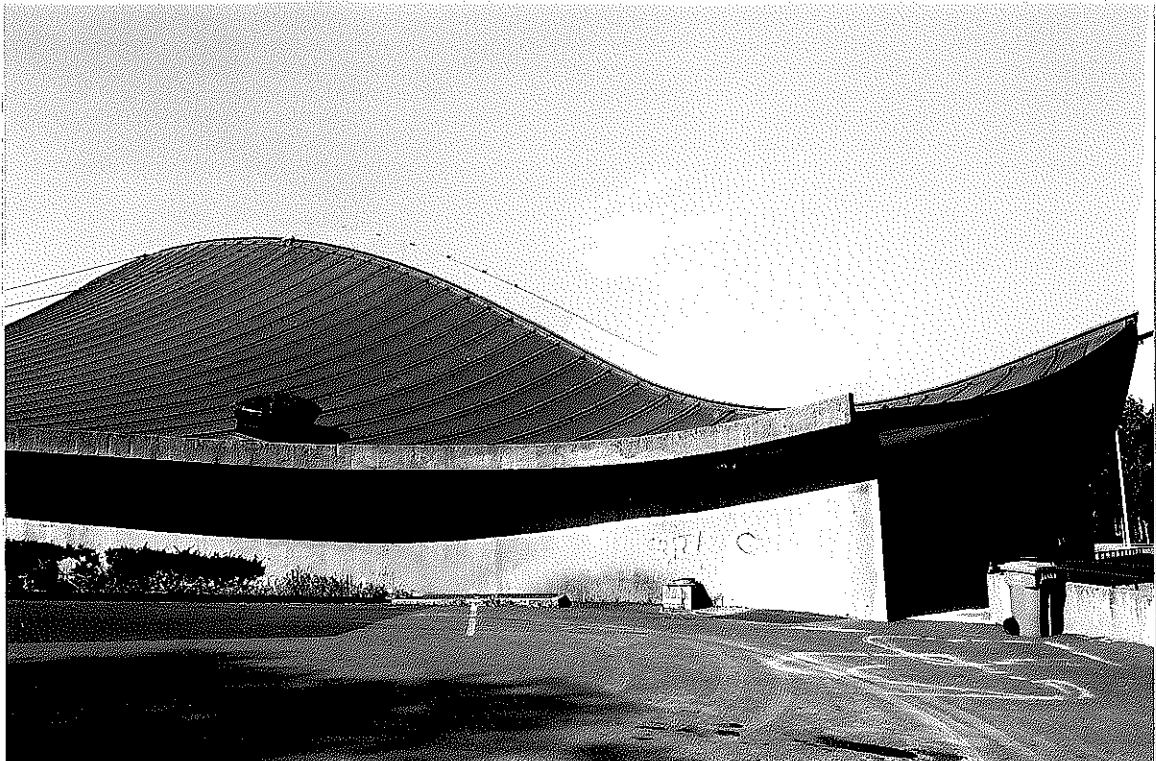
7. North end elevation, camera facing W
