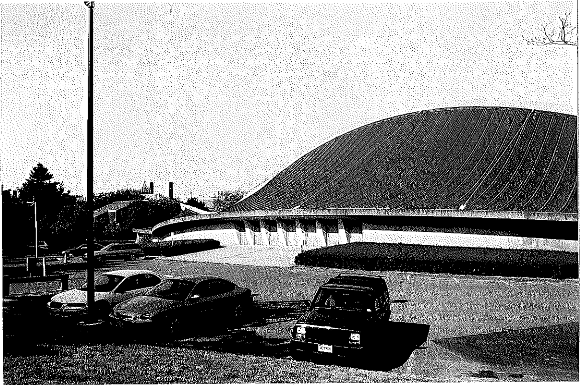
4. East elevation, camera facing SW
