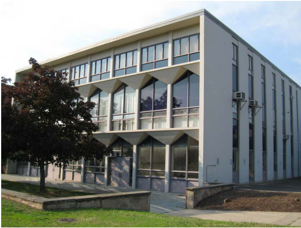
1. South (front) and east (side) elevations, camera facing northwest.
