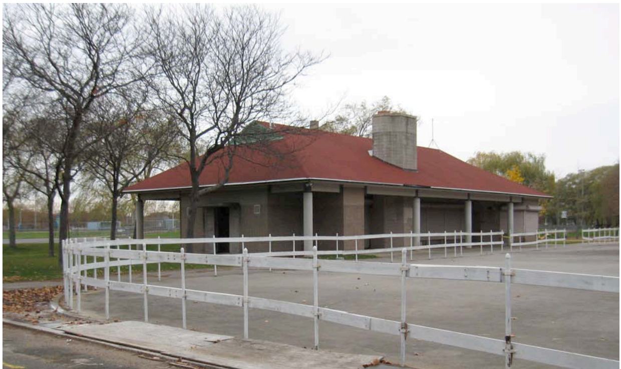
2. Southeast view of rink and building, camera facing northwest.
