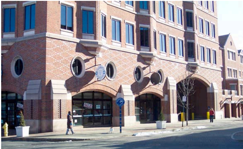
2. South detail view of Audubon Street façade, garage entry at right, camera facing east.
