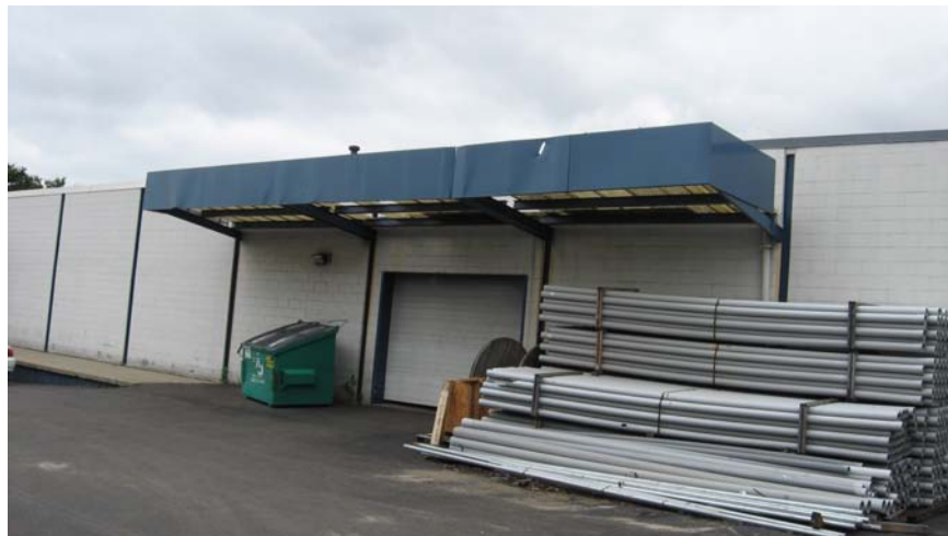
3. Detail of loading zone, east (front) elevation, camera facing southwest.
