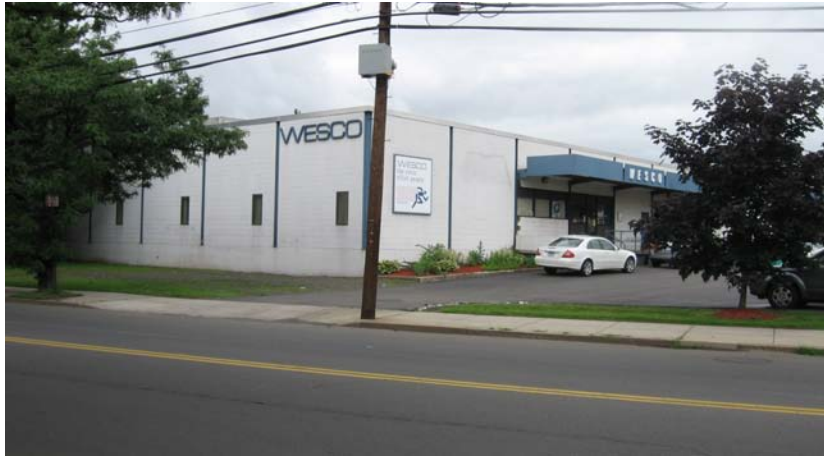
1. South (side) and east (front) elevations from Grand Avenue, camera facing northwest.
