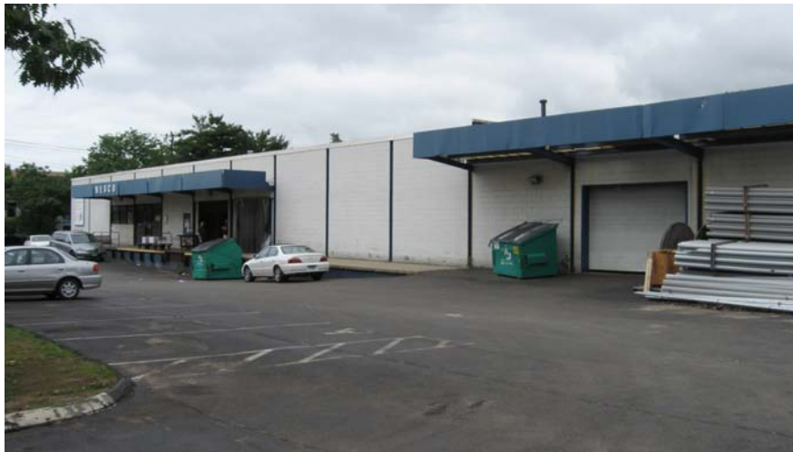
2. East (front) elevation from Wallace Street, camera facing southwest.
