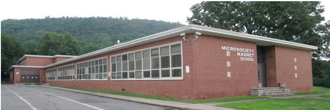
1. Southwest view of west classroom wing, camera facing north.
