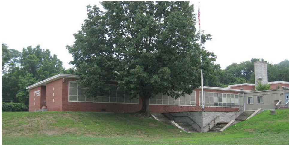
2. East view of west classroom wing, camera facing west, shows flagpole terrace, stone walls and steps down to play fields.
