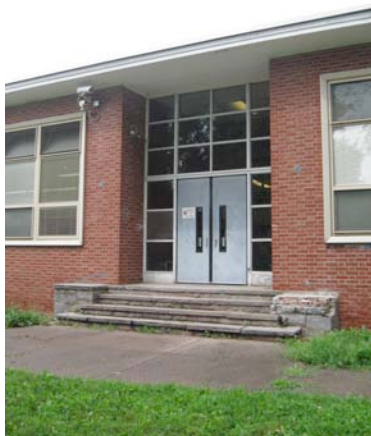
5. a. East doors, showing original frames and glazing
