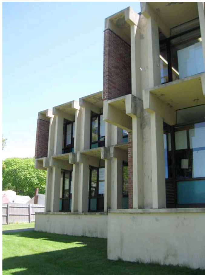
3. Detail view of northwest corner, camera facing northeast.
