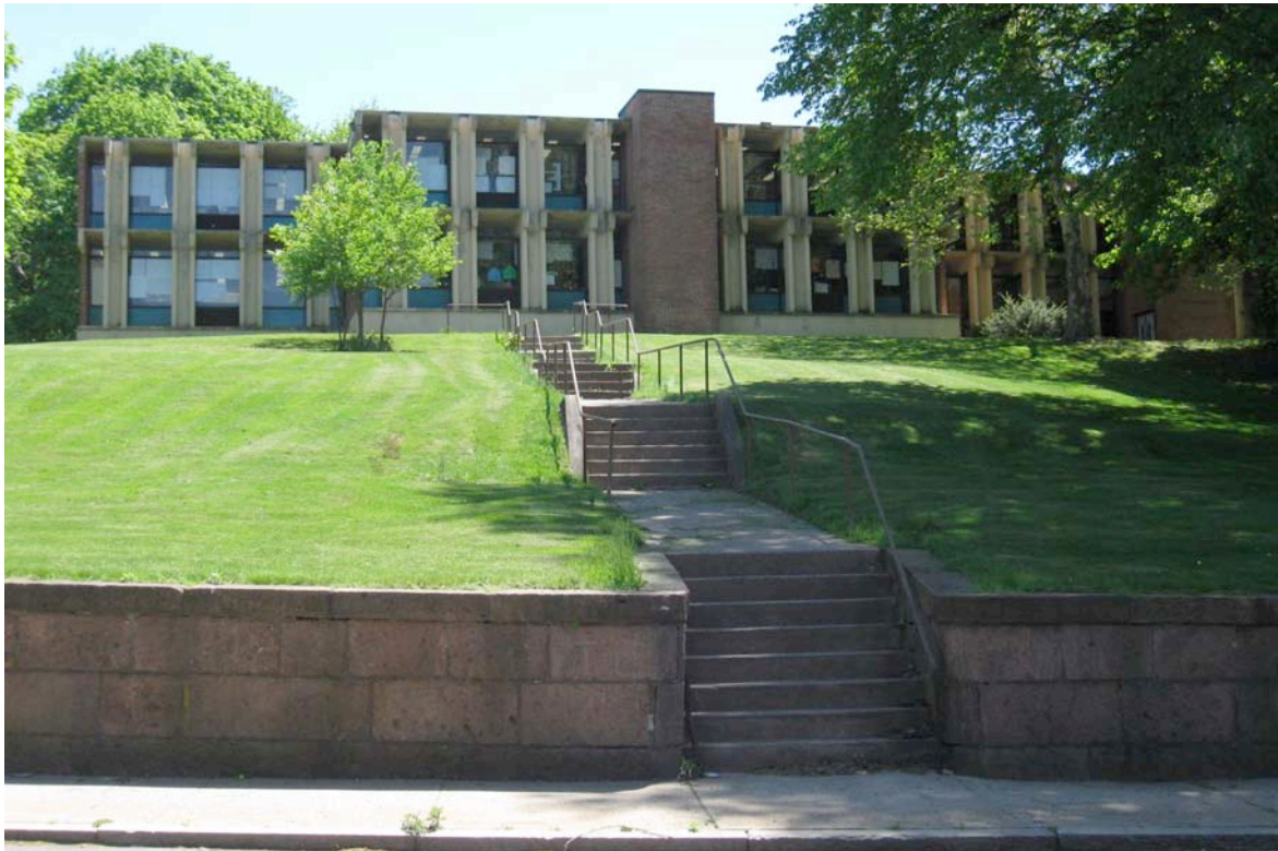
1. East view from Quinnipiac Avenue, camera facing west; wall and steps remain from previous school building.
