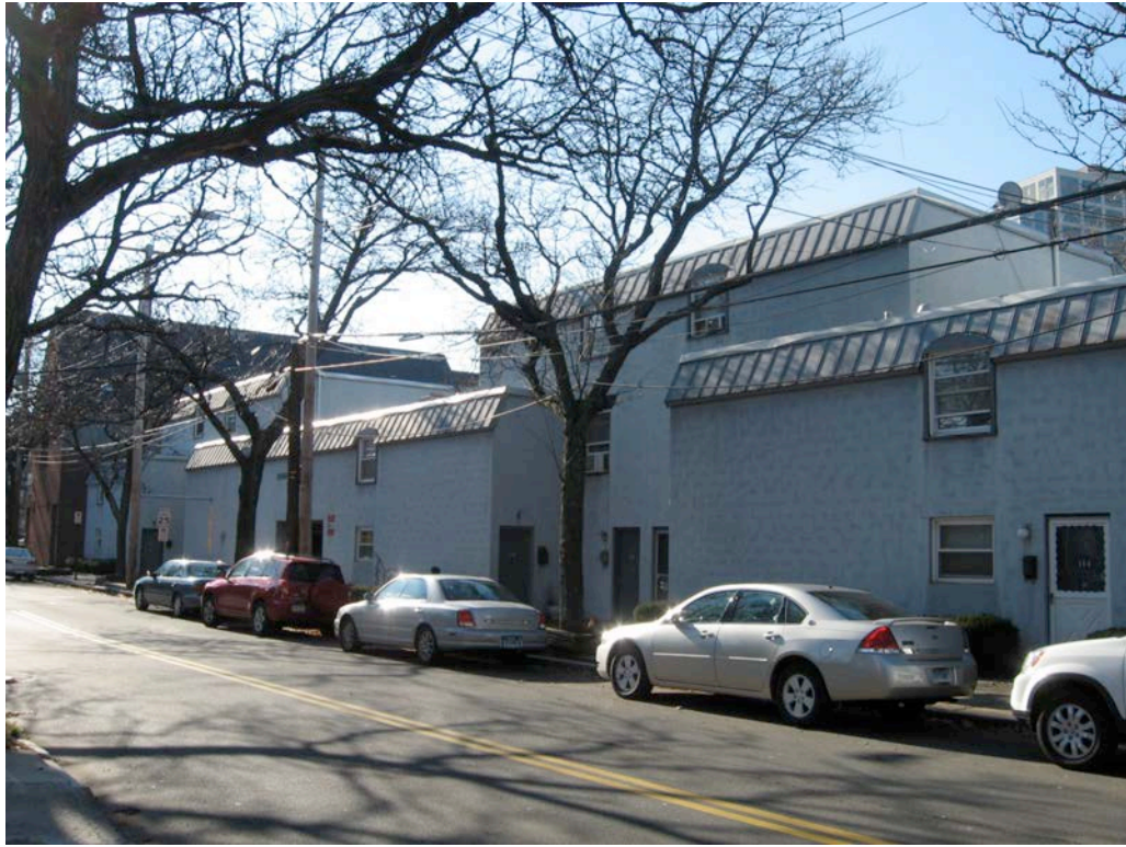
1. East (front) elevation from Olive Street, camera facing southwest.
