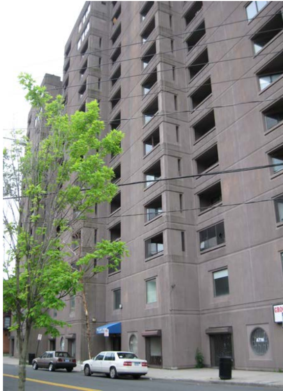
1. East view from Howard Avenue, camera facing southwest.
