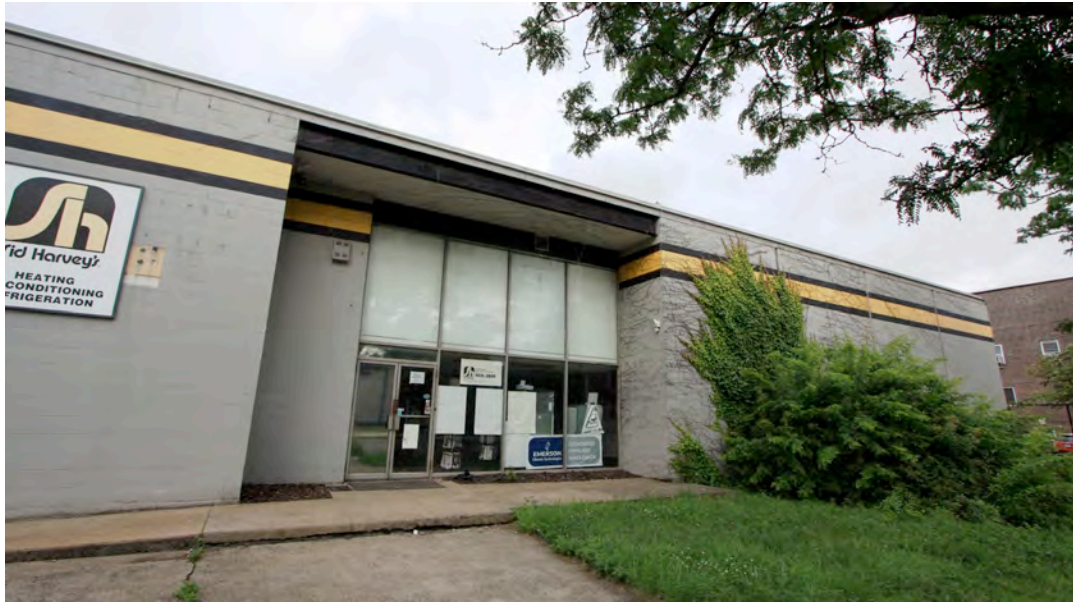
1. West view from Hamilton Street, camera facing east.
