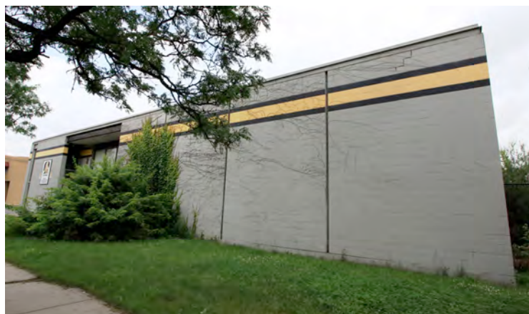
3. Southwest view from sidewalk, camera facing northeast.
