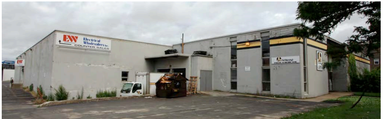
2. Northwest view from rear parking, camera facing southeast.
