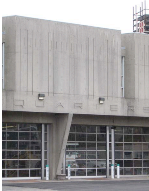
3. North elevation detail showing glazing, concrete detailing, signage.
