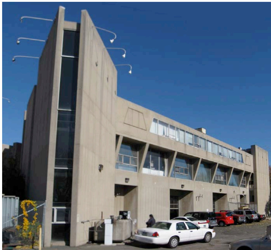
2. South elevation from rear parking area, camera facing north.
