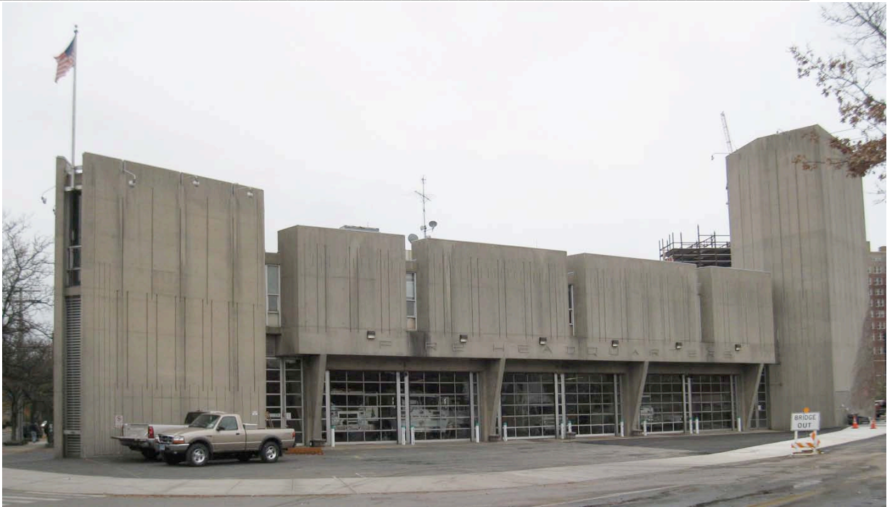
1. North elevation from the corner of Grand Avenue and Olive Street, camera facing south.
