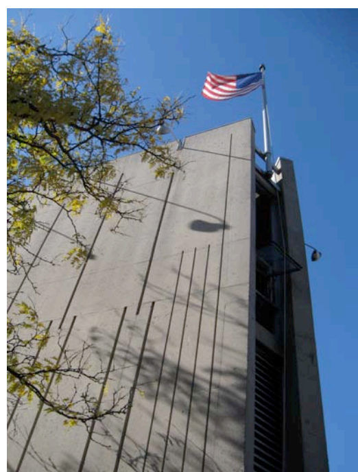
7. Detail of Northeast tower with Concrete Details
