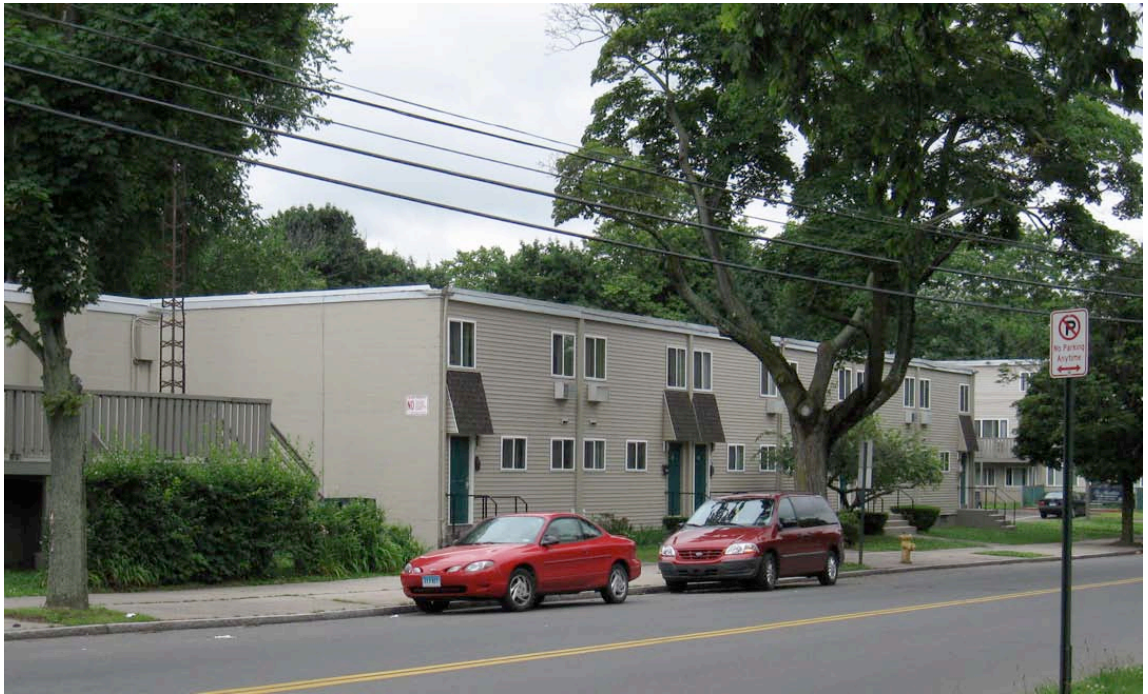
1. North elevation of street entry facade, duplex units; view from Goffe Street, camera facing southwest.
