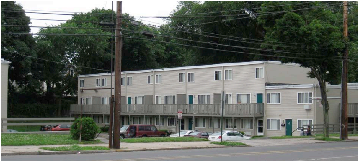
2. Rear elevation of Duplex-over-flat building type, camera facing southwest from Goffe Street.
