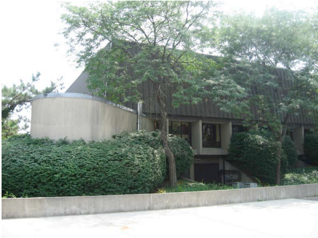
3. North (front) and east (side) elevations from the pedestrian walkway over Fitch Street, camera facing southwest.
