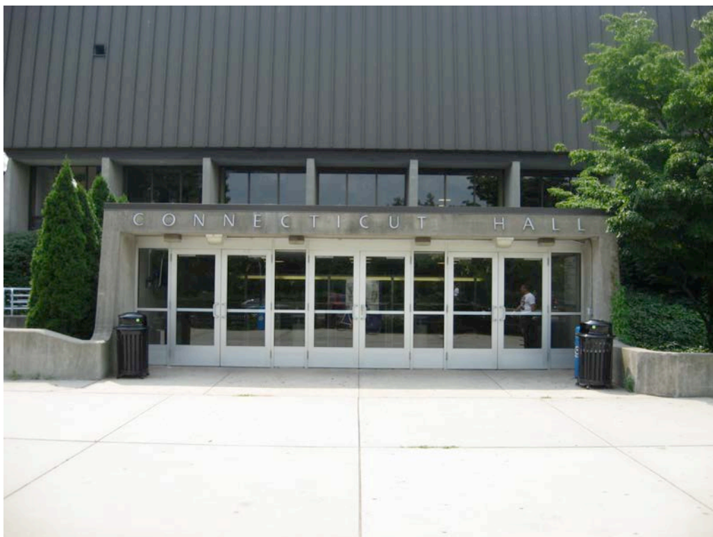
4. Detail of entry, camera facing south.
