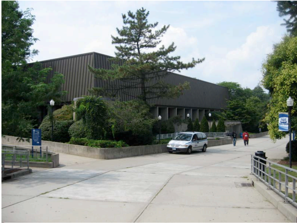
1. North (front) and east (side) elevations from the pedestrian walkway over Fitch Street, camera facing southwest.
