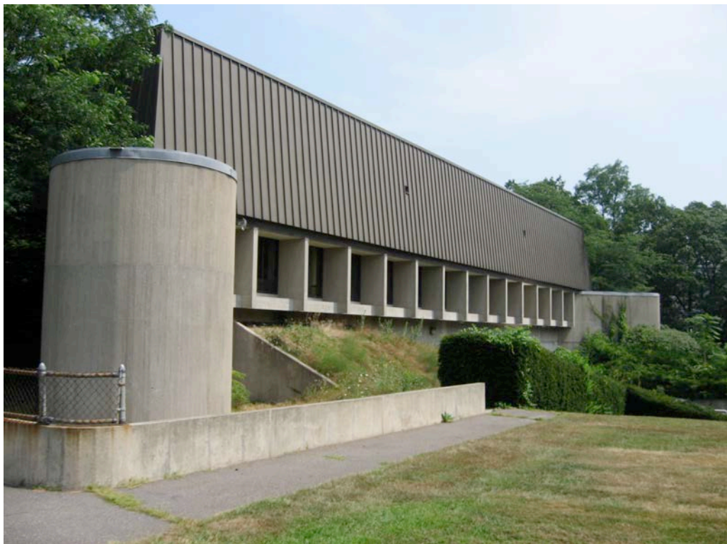
2. South (rear) elevation from Farnham Avenue, camera facing northeast.
