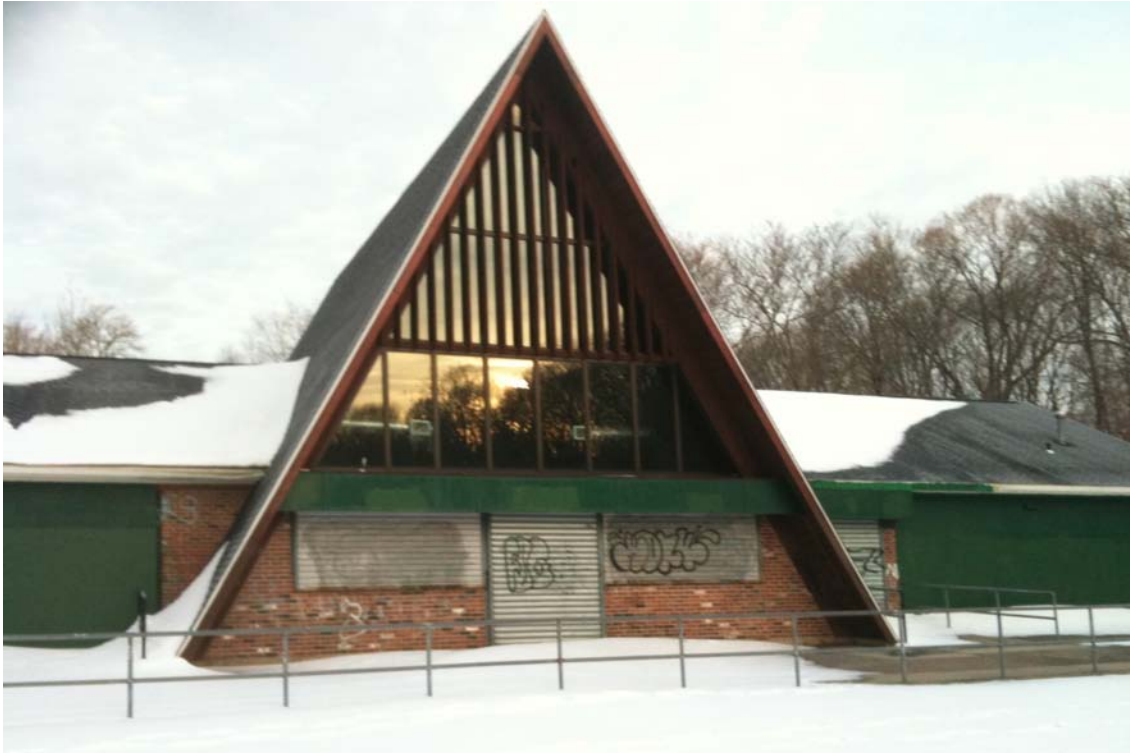
2. South detail view, camera facing north.
