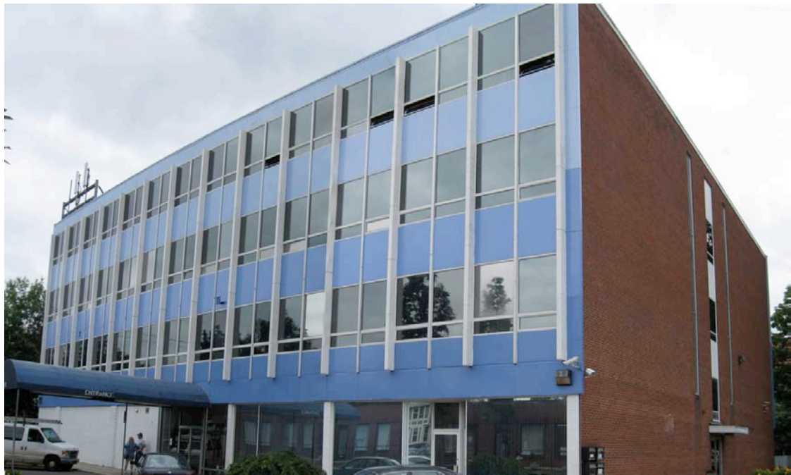
2. Northeast view from rear parking, camera facing southwest.
