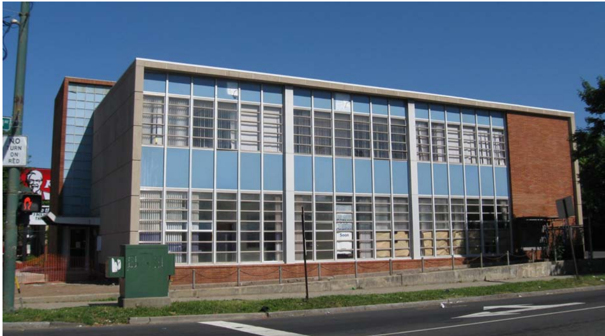
5. East view, camera facing west.
