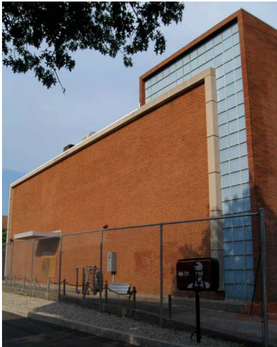
3. West elevation, camera facing northeast.
