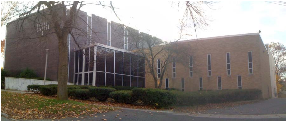
2. East and north sides viewed from West Prospect St., camera facing southwest.
