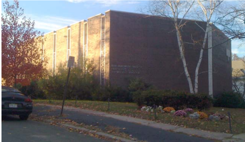
1. South and east facades viewed from Fairfield Street, camera facing north.
