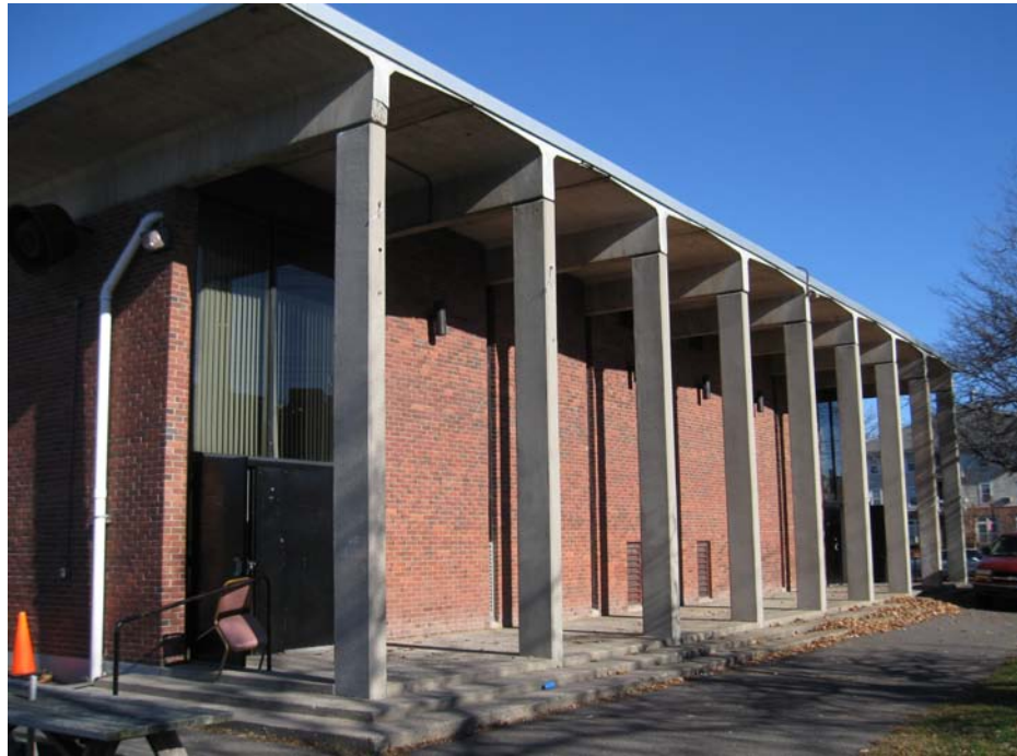
1. Southwest view from Webster Street, camera facing northeast.
