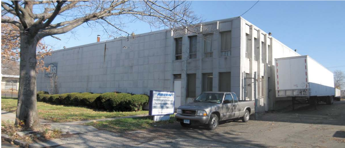
1. Southwest view of Wallace Street elevation, camera facing northeast.
