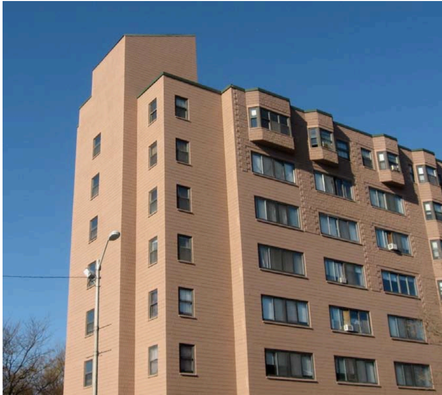
2. East (front) and south (side) elevations from Union Avenue, camera facing northwest.
