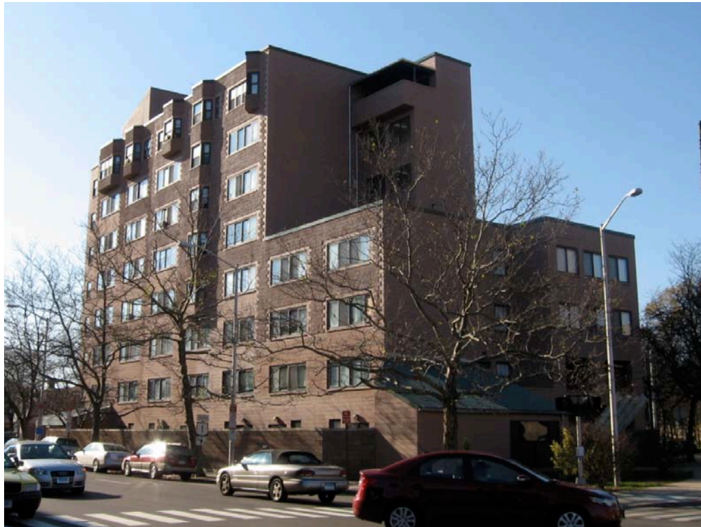
1. East (front) and north (side) elevations from Union Avenue, camera facing southwest.
