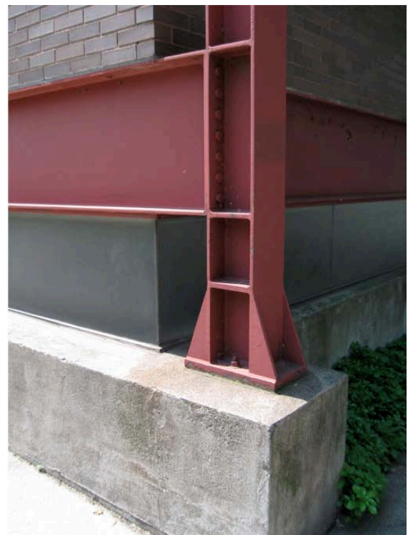
5. Corner detail of structural steel.
