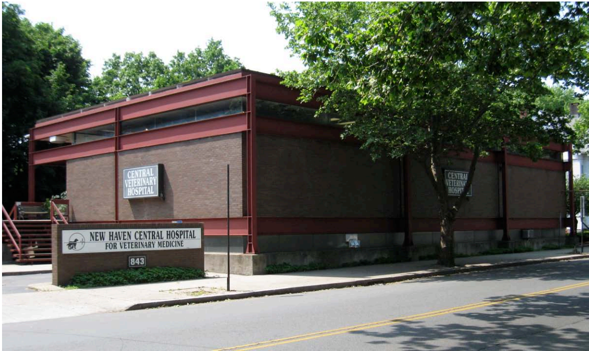
1. North view from State Street, camera facing south.
