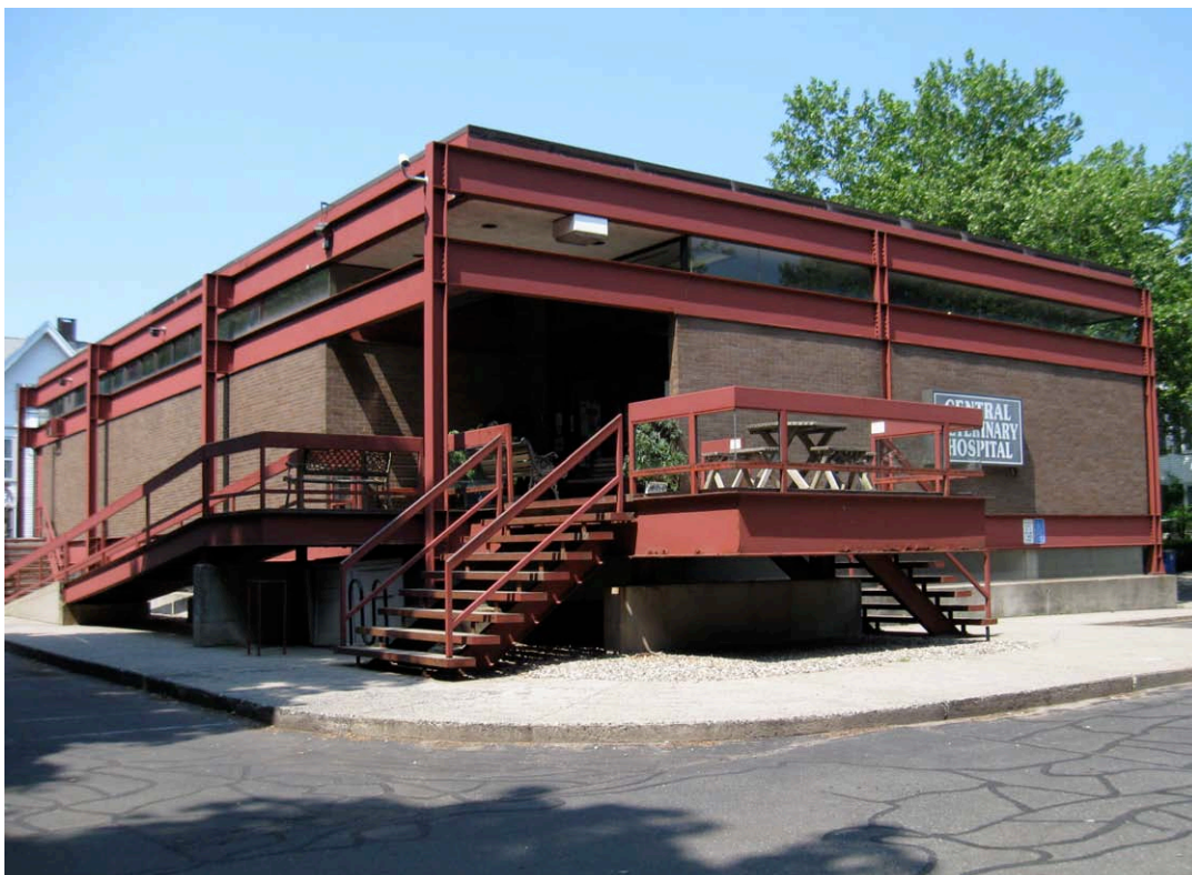
2. East view of entry porch from rear parking, camera facing west.
