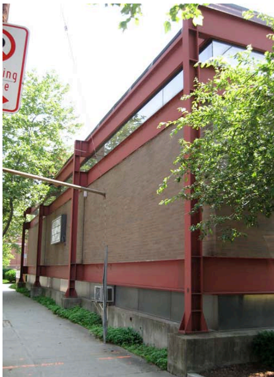
4. West view - street facade.
