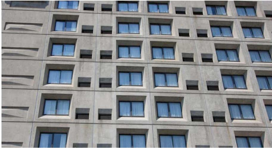
3. East detail view from parking, camera facing west.
