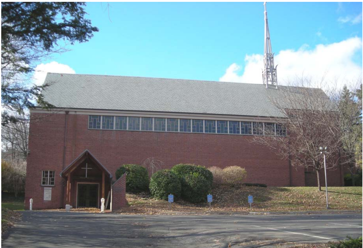
3. East view of sanctuary wing, camera facing west.
