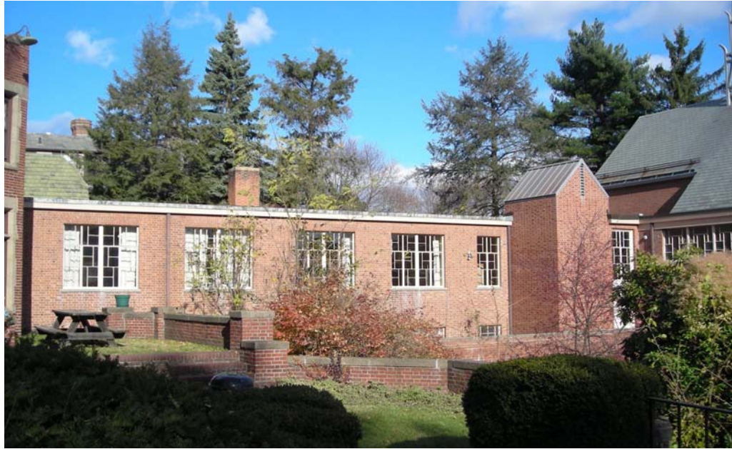
2. South view of education wing, camera facing north.
