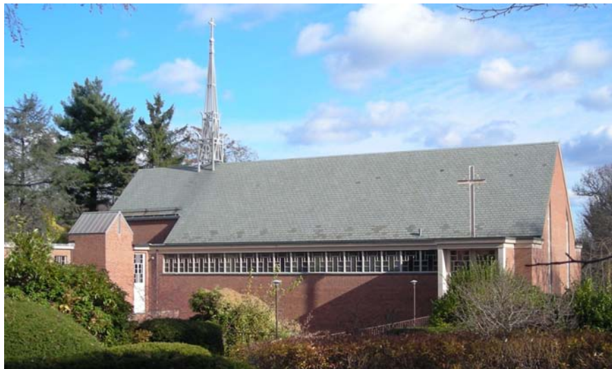
1. Southwest view of sanctuary, camera facing northeast.
