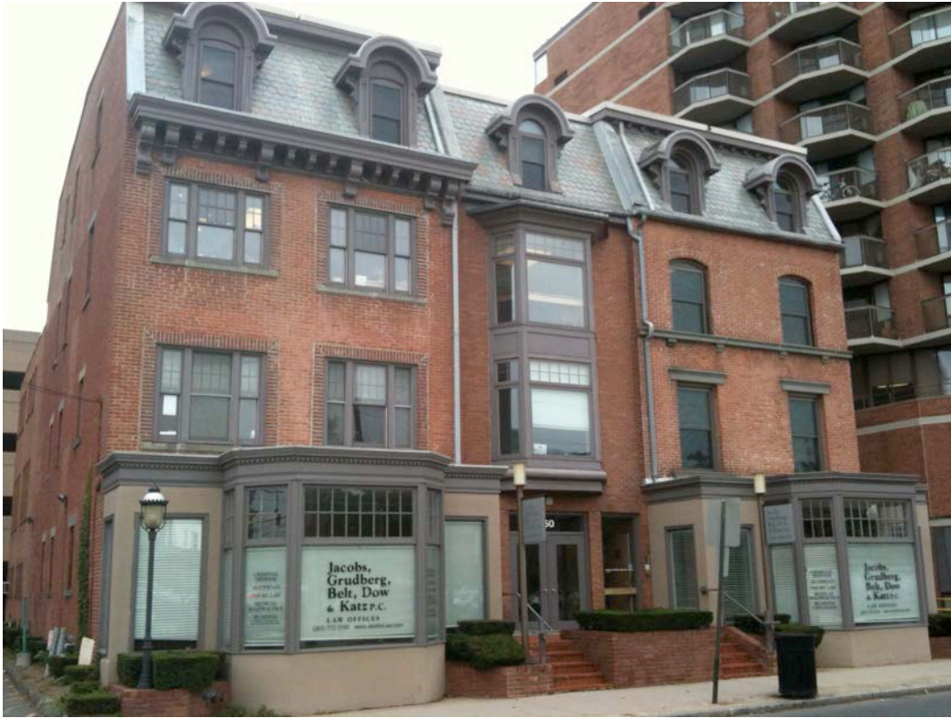
1. Southeast view from Orange Street, camera facing northwest.
