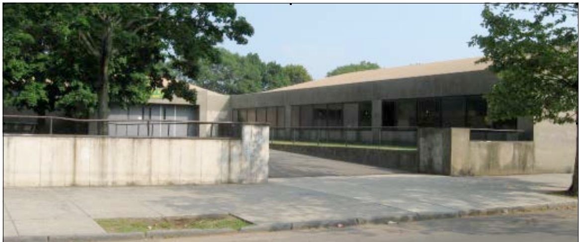
3. North view from Nash Street, camera facing south.
