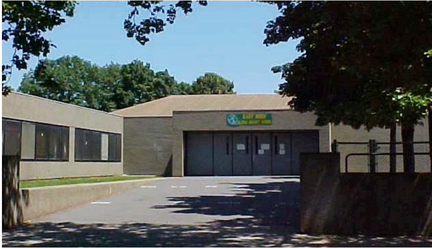
1. Northwest view from Nash Street, camera facing southeast.
