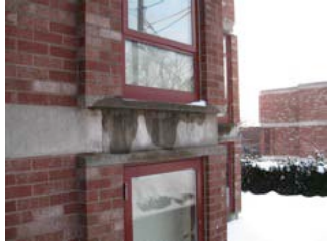
3. Detail of concrete belt course and window bay.
