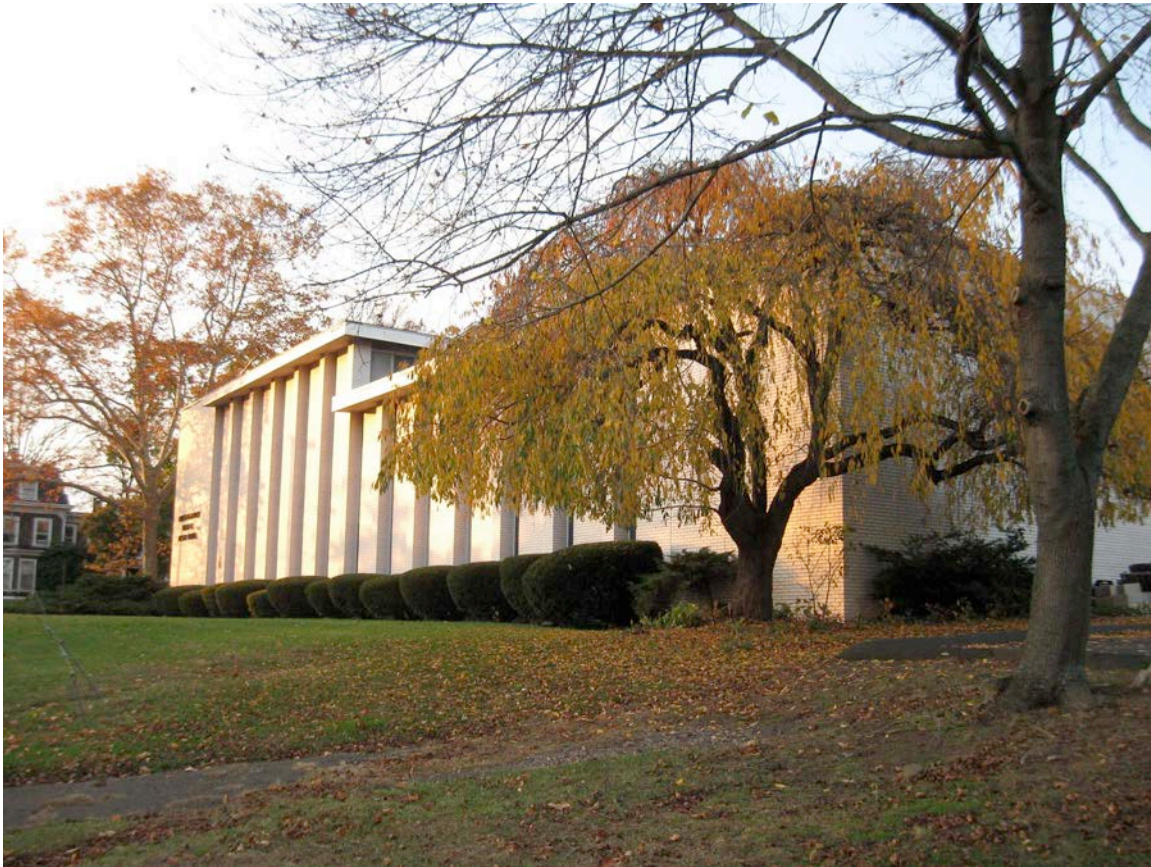
2. Southwest view from Whalley Avenue, camera facing northwest.
