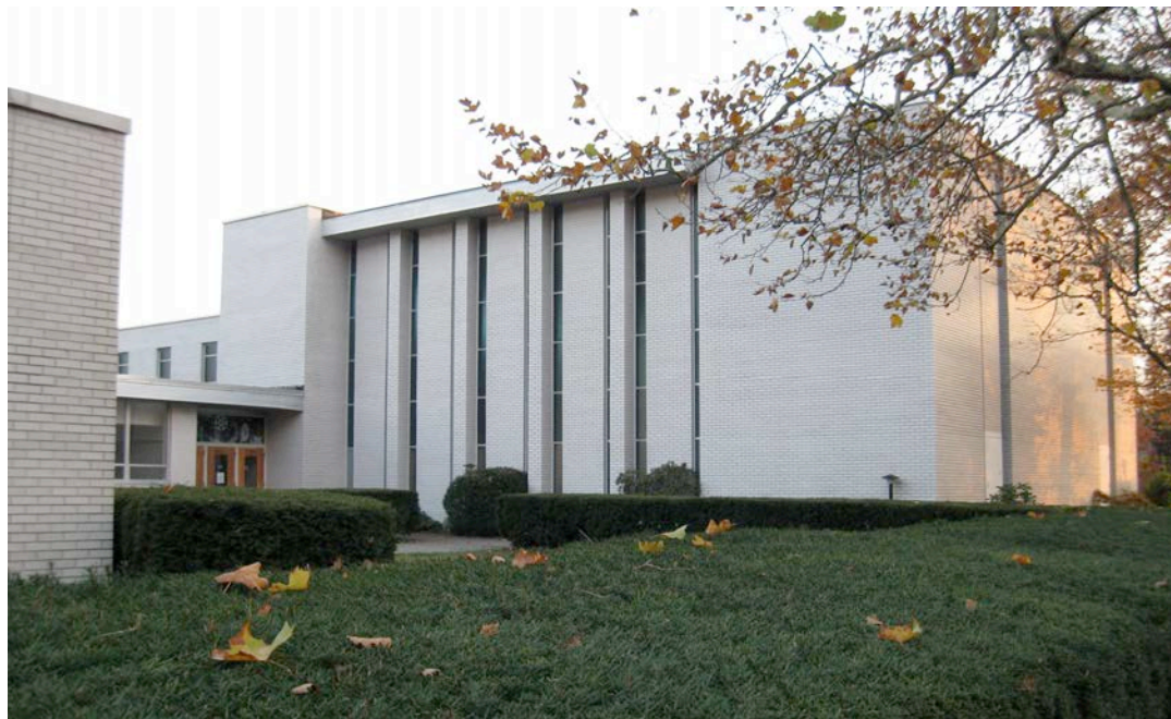
3. Northwest view from Harrison Street, camera facing southeast.
