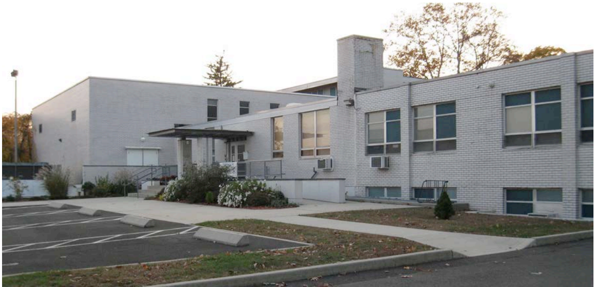
4. Northeast (rear) view, camera facing southeast.
