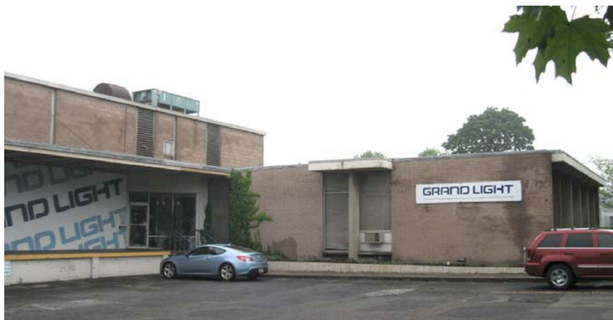
6. Southeast view of the office wing (right) and warehouse with contractor entrance (left), camera facing north.
