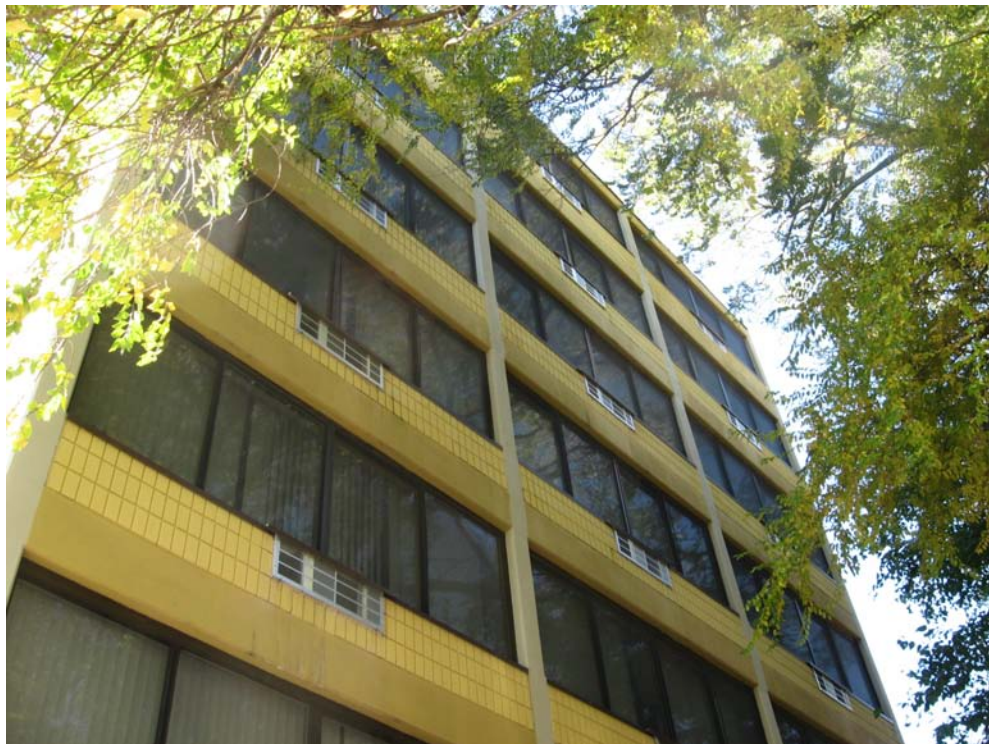
2. North (rear) elevation from parking lot on east side of building, camera facing southwest.
