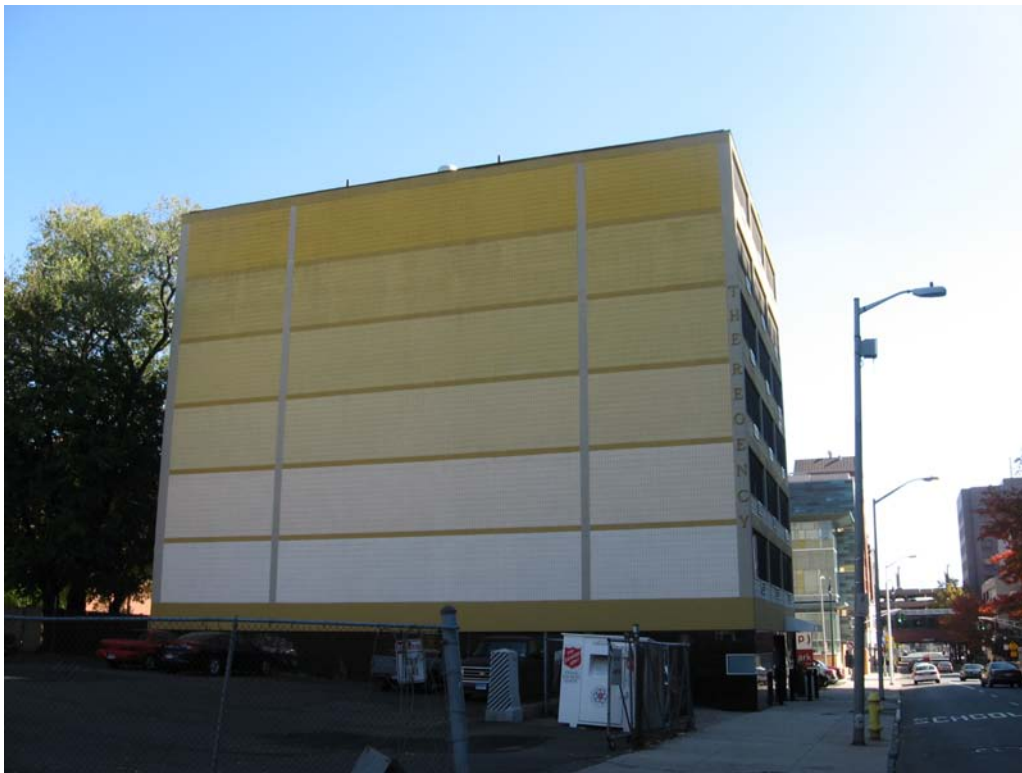
1. West (side) and south (front) elevations from George Street, camera facing east.
