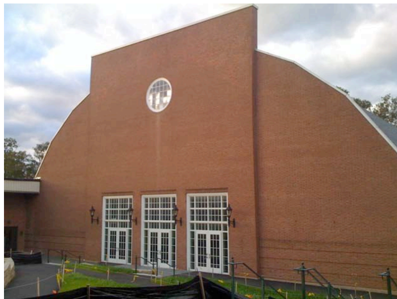
2. Southeast view of south facade, camera facing northwest
