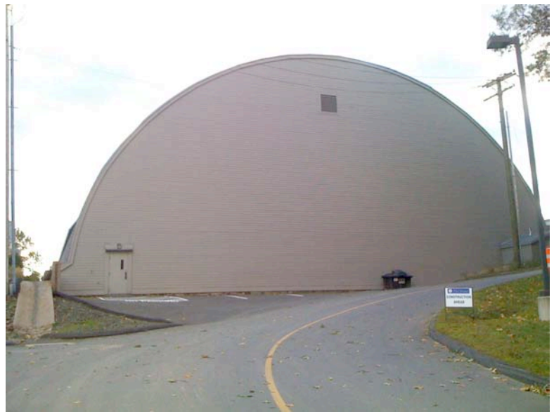
6. North (rear) elevation, camera facing south
