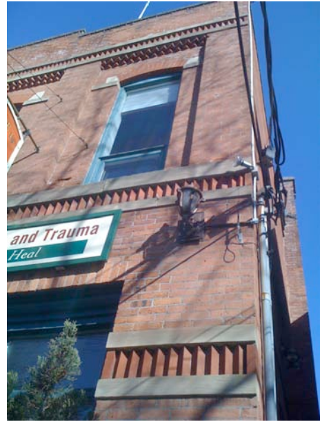
3. Detail view of southwest (front) facade.
