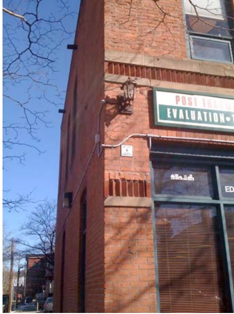
2. Detail view of southwest (front) facade.
