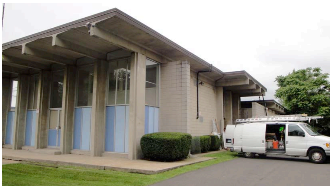
2. North and east elevations, camera facing southwest.
