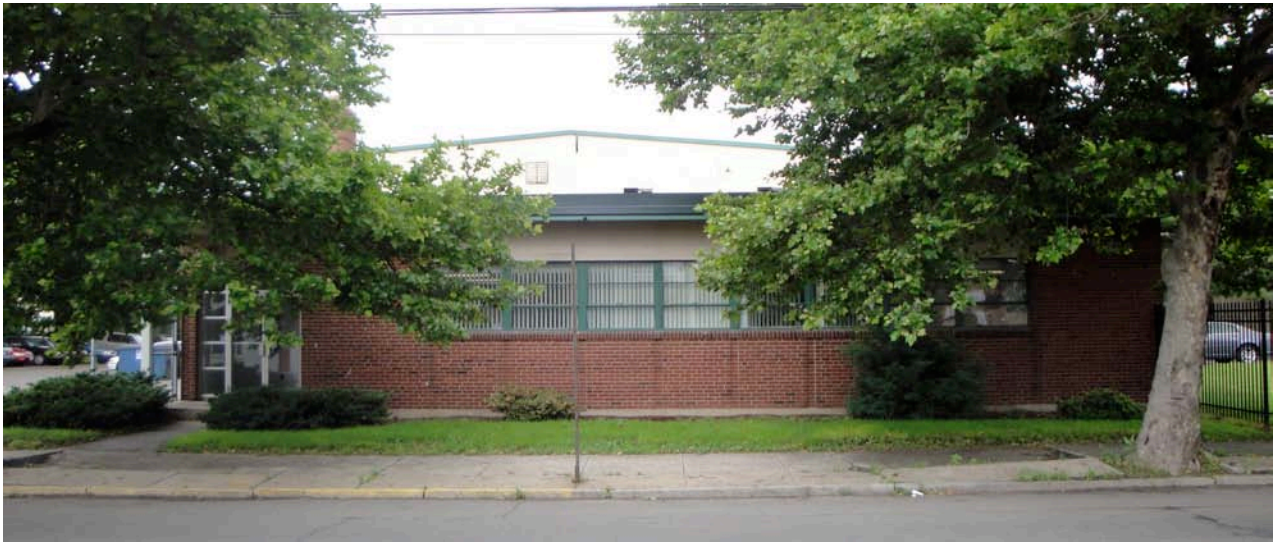
1. East view from street, camera facing west.
