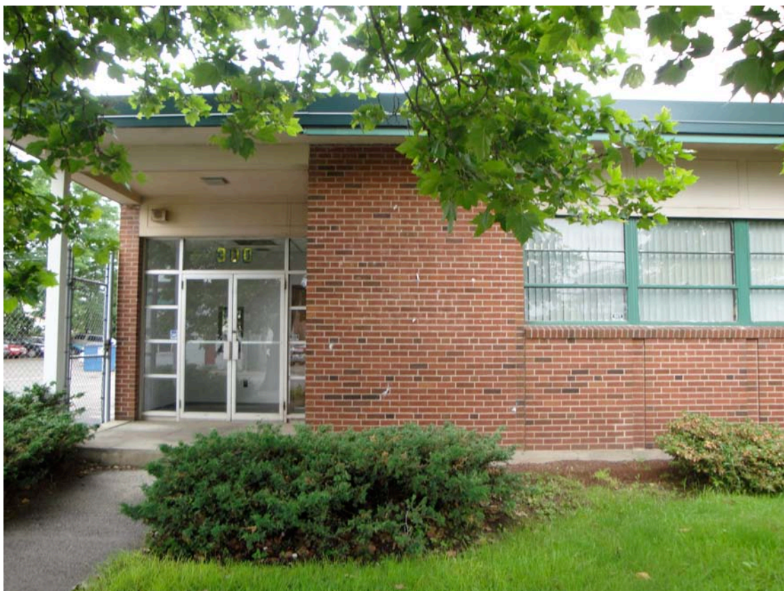
2. East detail view of entrance, camera facing west.
