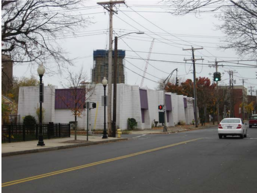
1. West (front) and north (side) elevations from Dixwell Avenue, camera facing southeast.
