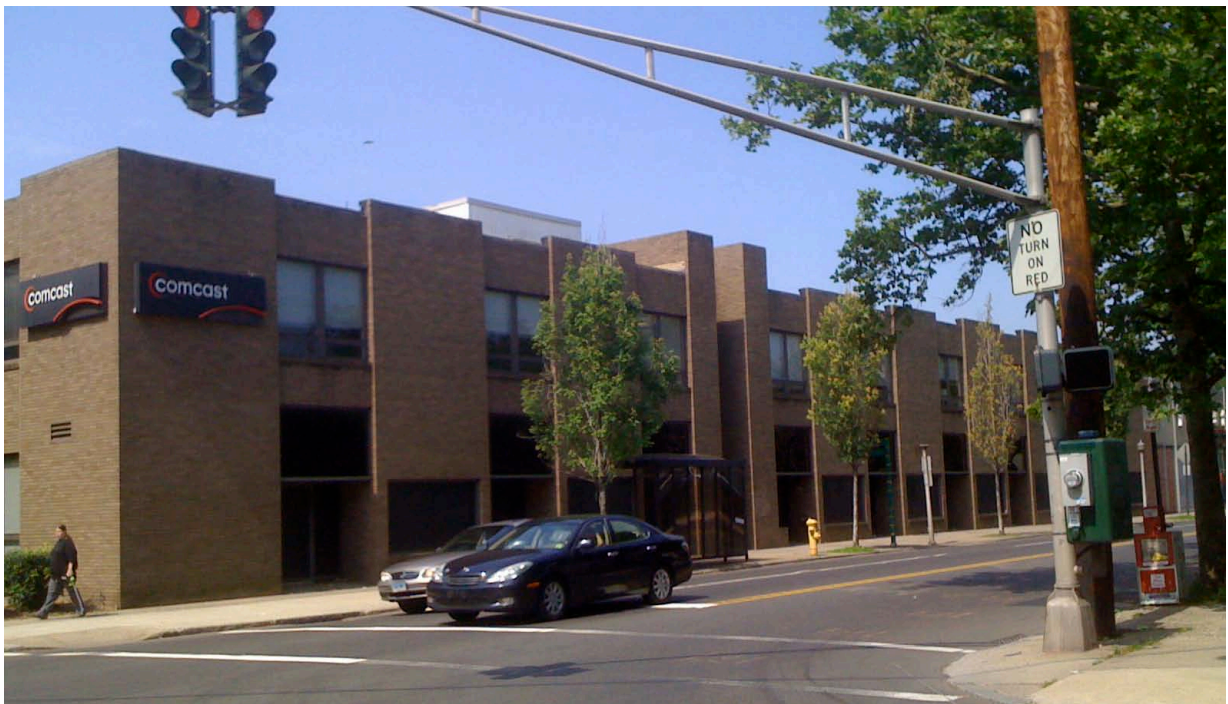
3. View of north facade along Chapel Street, camera facing southwest.
