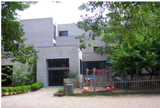
2. Rear Courtyard and South Elevation, camera facing north.
