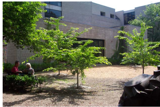
3. Rear Courtyard and South Elevation, Camera facing northeast.
