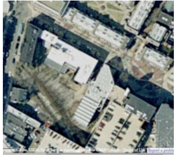
5. Aerial view from Google Maps; sawtooth skylights are visible on the rear portion of the roof.
