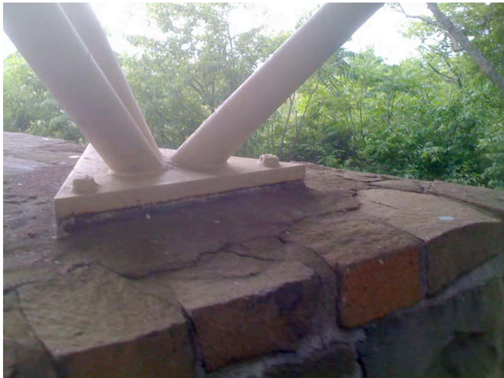
4. Detail of steel column base, camera facing west.
