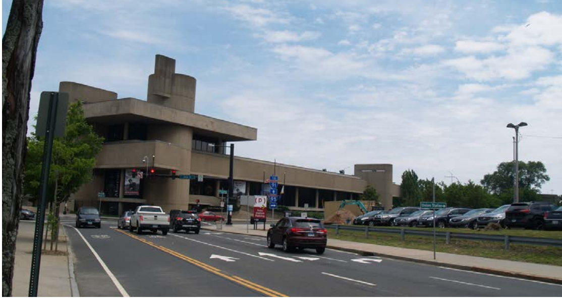
Photo 6. Northwest view of 1 State Street, camera facing southeast along George Street.
