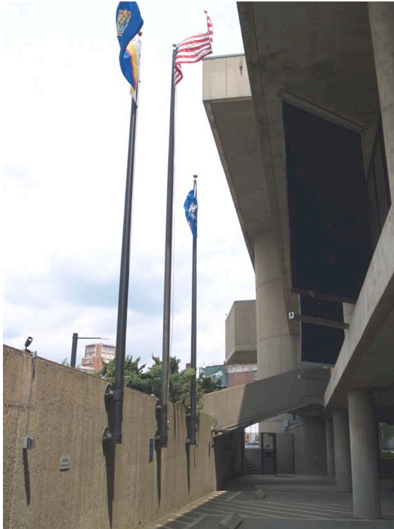
Photo 16. Lower level view of parking and side view of the entry stair, camera facing north, showing the relationship of the sunken parking level to street and first floor elevations.
