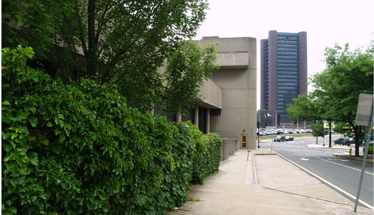
Photo 12. North view, camera facing west, showing the building corner with the Knights of Columbus headquarters at 1 Columbus Plaza in the distance beyond the former Coliseum site.
