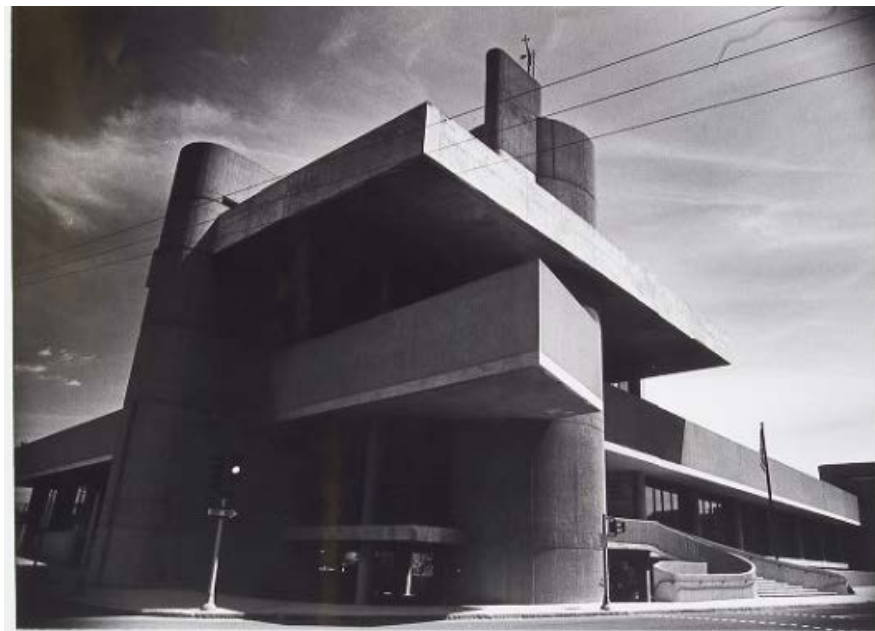
Photo 5. Northwest historical view of Community Services Building in 1971, camera facing southeast. New Haven Redevelopment Collection, New Haven Museum.
