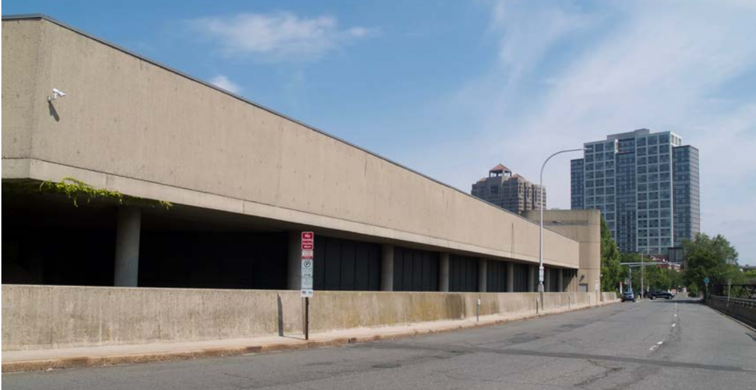
Photo 10. East view of 1 State Street, camera facing north.
