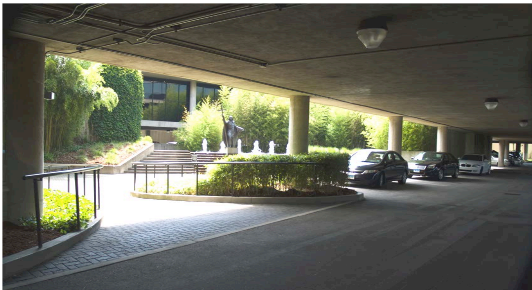
Photo 13. Lower level view of parking and courtyard, camera facing southeast.
