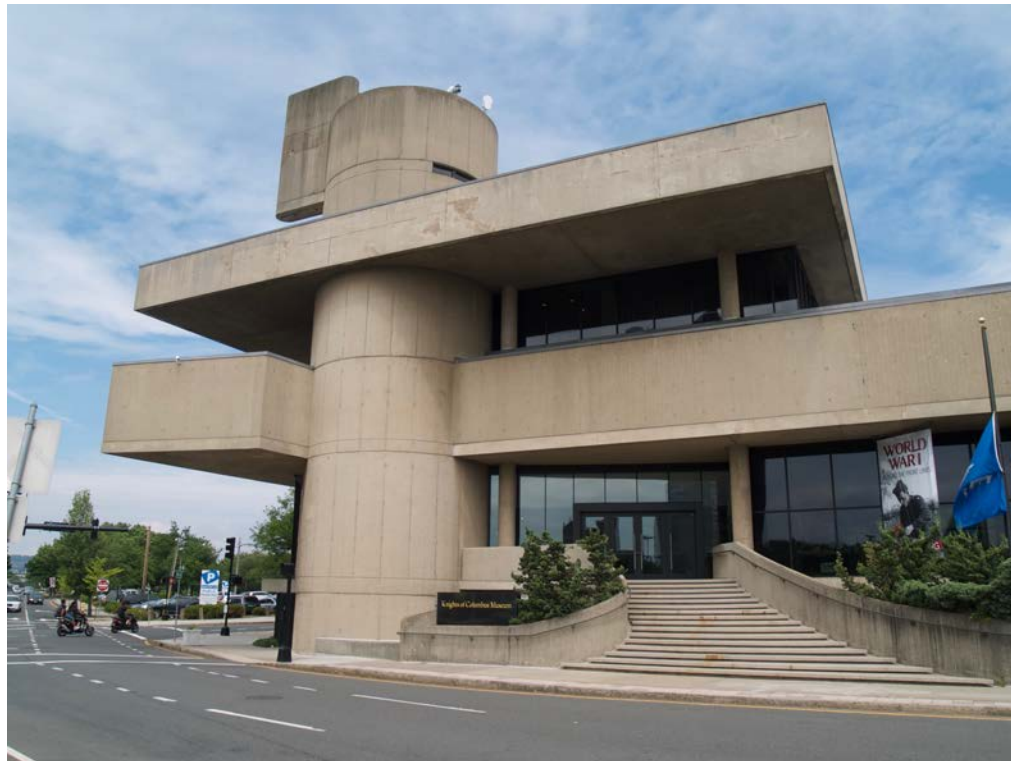
Photo 7. West detail view of 1 State Street, camera facing east, showing the main entrance and sculptural massing at the northwest corner.
