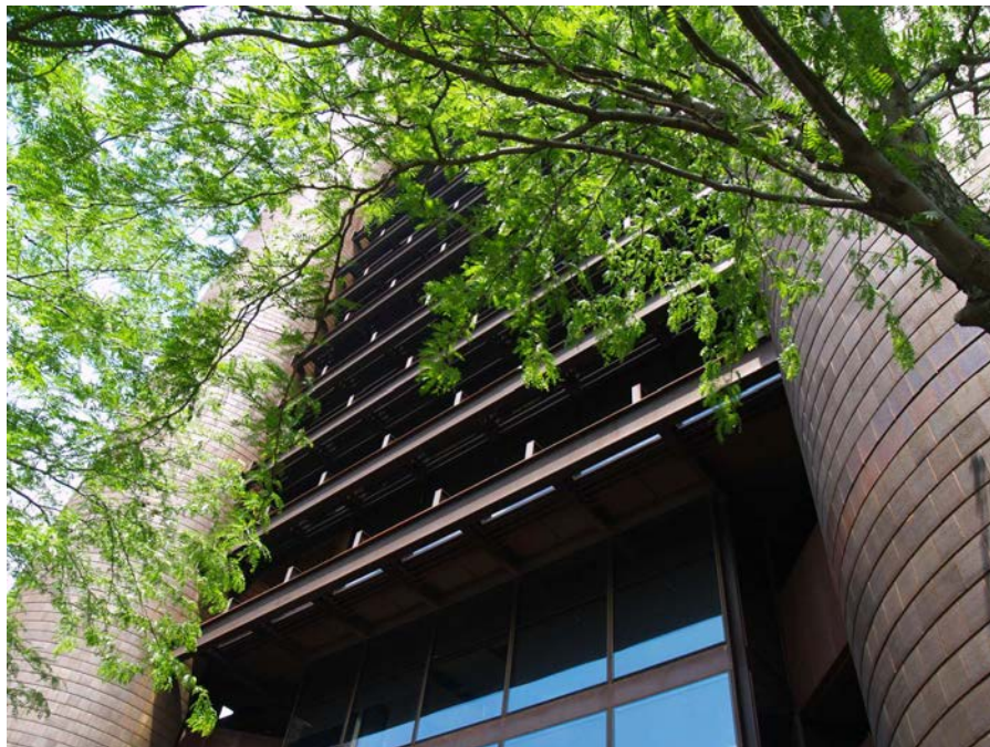
Photo 11. Detail southwest view of upper facade, camera facing north.
