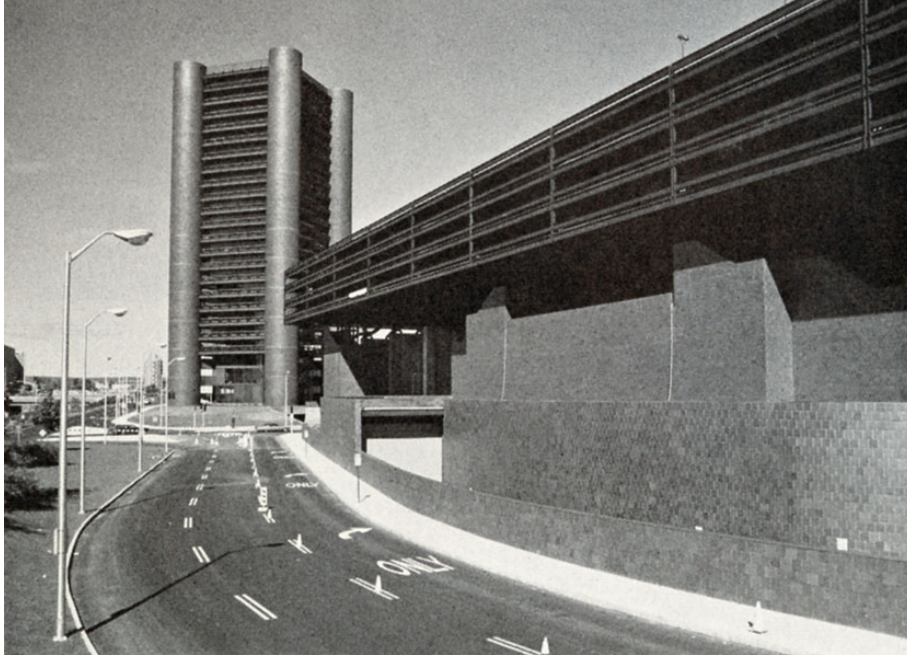
Photo 5. Southeast historical view of the New Haven Veterans Memorial Coliseum and 1 Columbus Plaza, Knights of Columbus Building; camera facing northwest. New Haven Redevelopment Collection, New Haven Museum.
