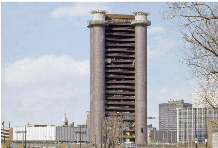
Photo 6. Southeast view of 1 Columbus Plaza during construction, camera facing northwest. Note the reinforced concrete corner pillars with masonry cladding partially installed. Photo courtesy of KRJDA, accessed 7/28/2017 at http://www.krjda.com/Images/KofC%20Images/KofC_16.jpg
