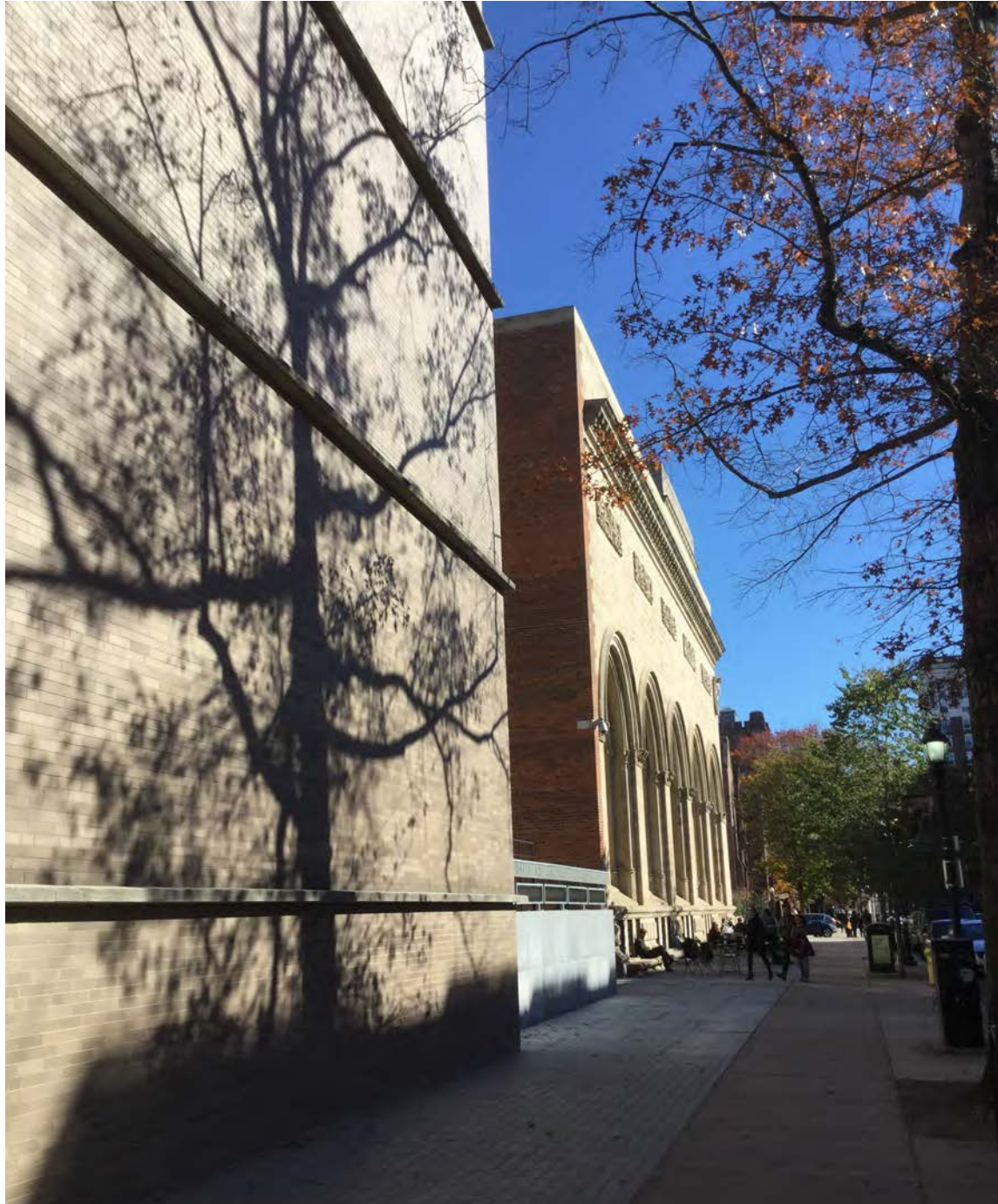
Photo 6. South view of Chapel Street façade with Louis Kahn Building in the foreground and Old Yale Art Gallery at rear; camera facing east.
