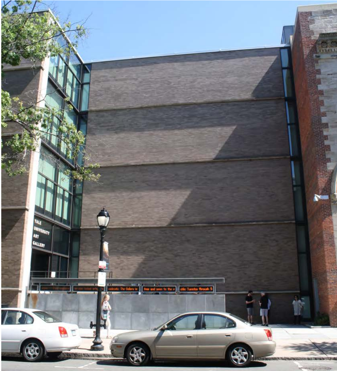
Photo 7. South view of Louis Kahn Building entry; camera facing north.
