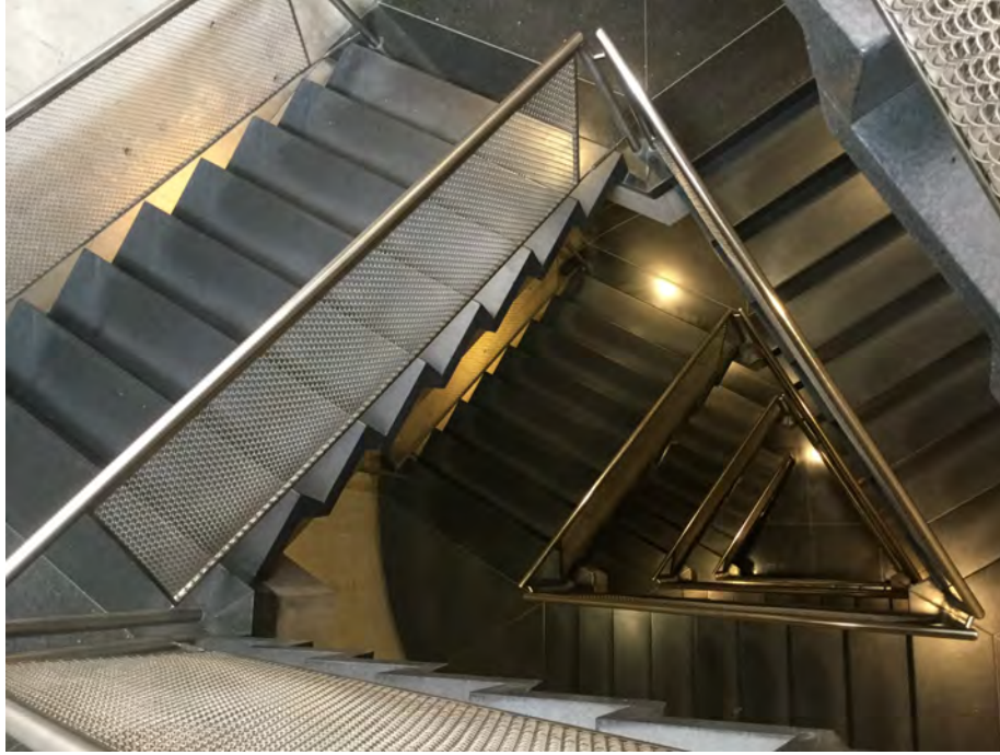
Photo 13. Interior view of Louis Kahn Building stairwell seen from the fourth floor; camera facing down.
