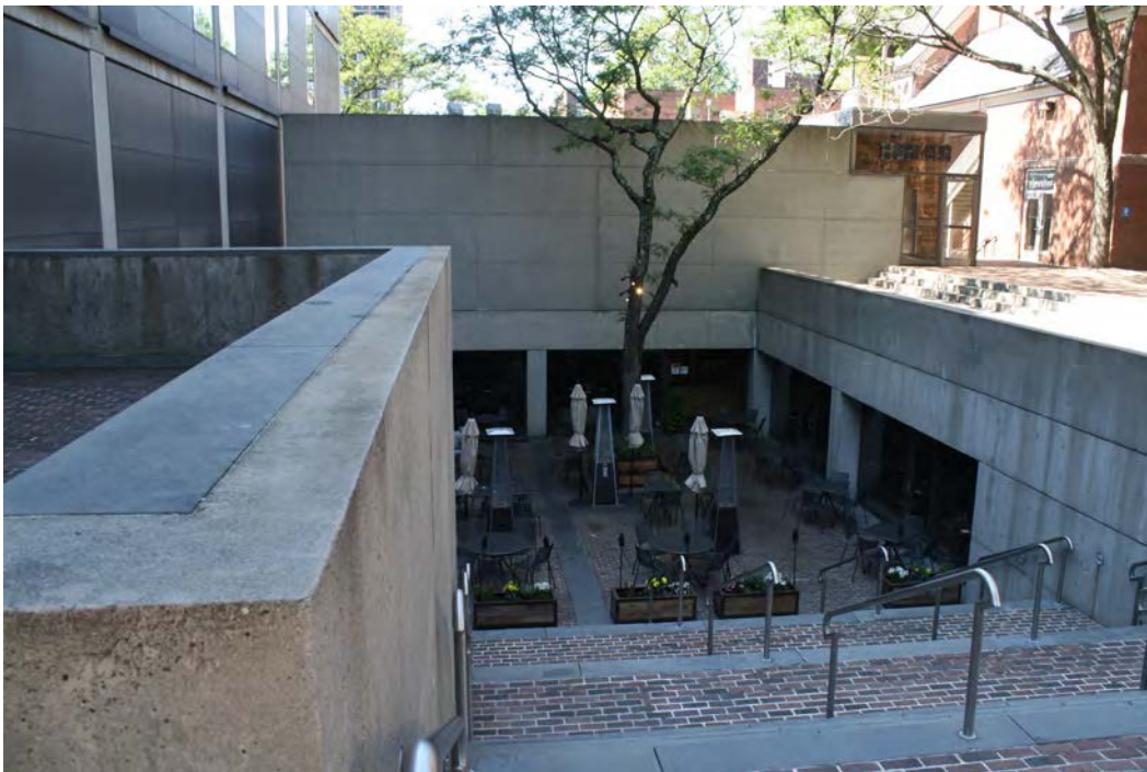
Photo 6. North view of the Lower Court; camera facing south. Elevator lobby for lower level is at right rear.
