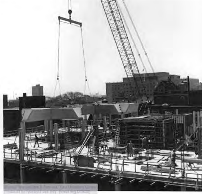
Photo 17. Construction photograph showing installation of skylight well “V-beams,” camera facing south. Image No. 3520. Construction of Yale Center for British Art. Louis Isadore Kahn collection, 19511978 (inclusive), 19621977 (bulk). MS 1345. Manuscripts & Archives, Yale University.
