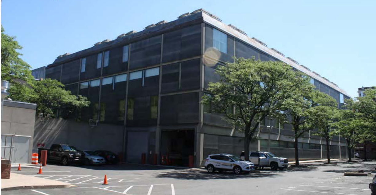
Photo 5. Southwest view, camera facing northeast, showing loading dock and parking.
