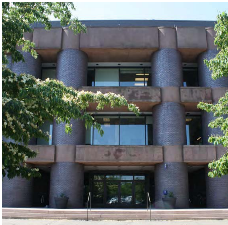
Photo 6. North detail view of Kline Geology Laboratory entrance; camera facing south.
