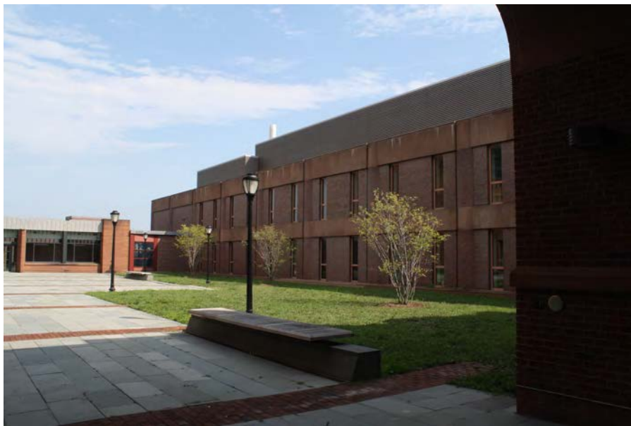
Photo 10. North view of Kline Chemistry Laboratory; camera facing southeast. An enclosed courtyard is formed by the Class of 1954 Chemistry Research Building on three sides and the Kline Chemistry Laboratory building on the south.
