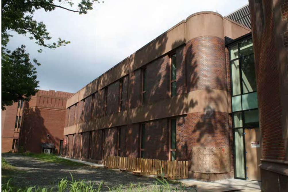
Photo 9. West view of Kline Chemistry Laboratory; camera facing northeast. At right is the Sterling Chemistry Laboratory, at far left is the Class of 1954 Chemistry Research Building.
