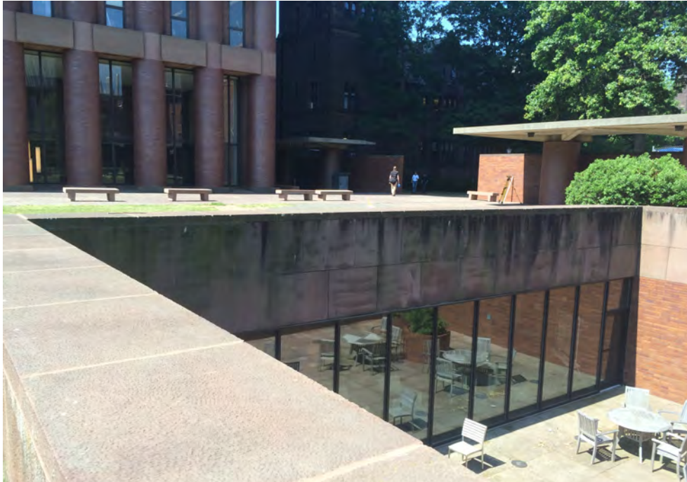
Photo 17. North view of Kline Biology Tower lower level courtyard; camera facing southwest.
