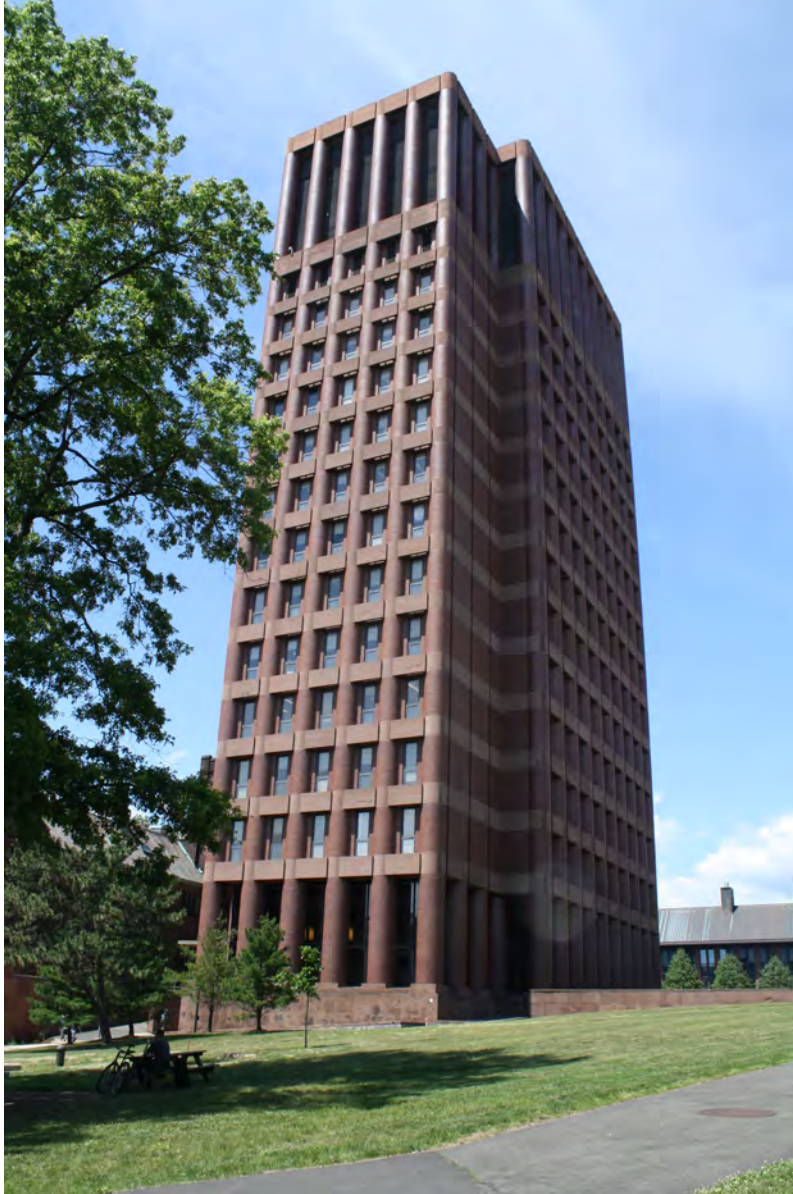
Photo 13. Southeast view of Kline Biology Tower; camera facing northwest.
