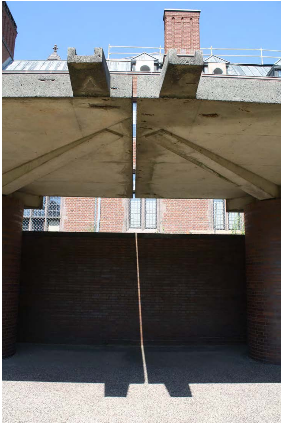
Photo 19. View of west side of colonnade; camera facing west.
