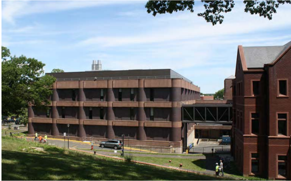
Photo 5. West view of Kline Geology Laboratory; camera facing east.
