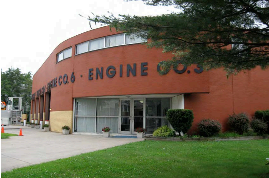
Photo 5. West detail view of entrance, camera facing east.
