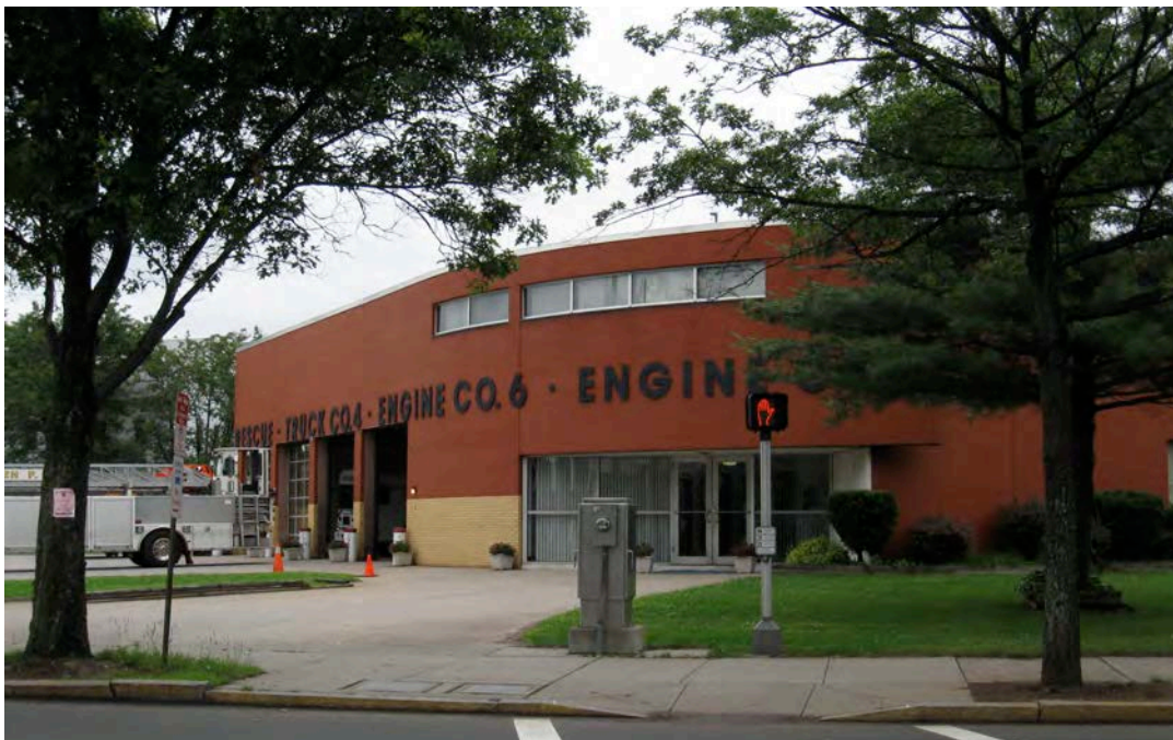
Photo 4. West view of 125 Goffe Street, camera facing east.
