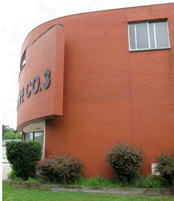
Photo 6. Southwest view of façade with cantilevered wall; camera facing north.
